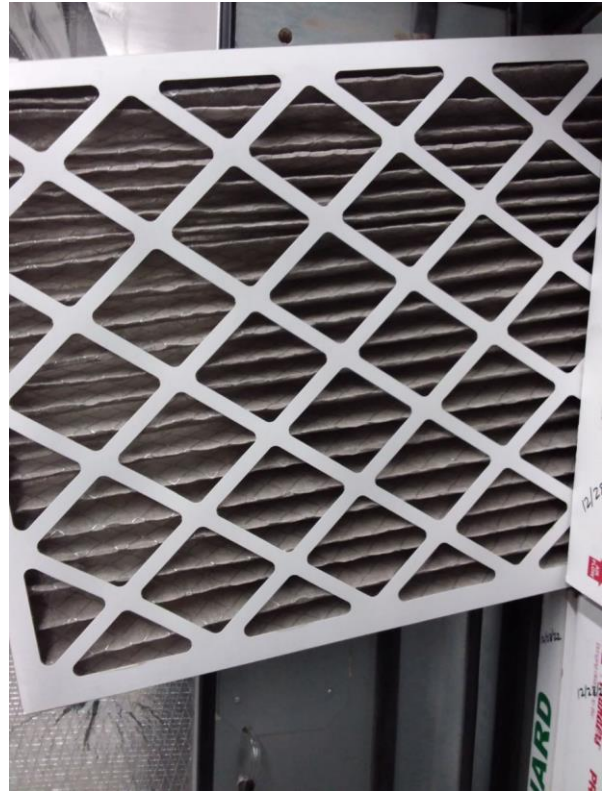
AHU10 Mixed Pre-Filter Cleanliness
