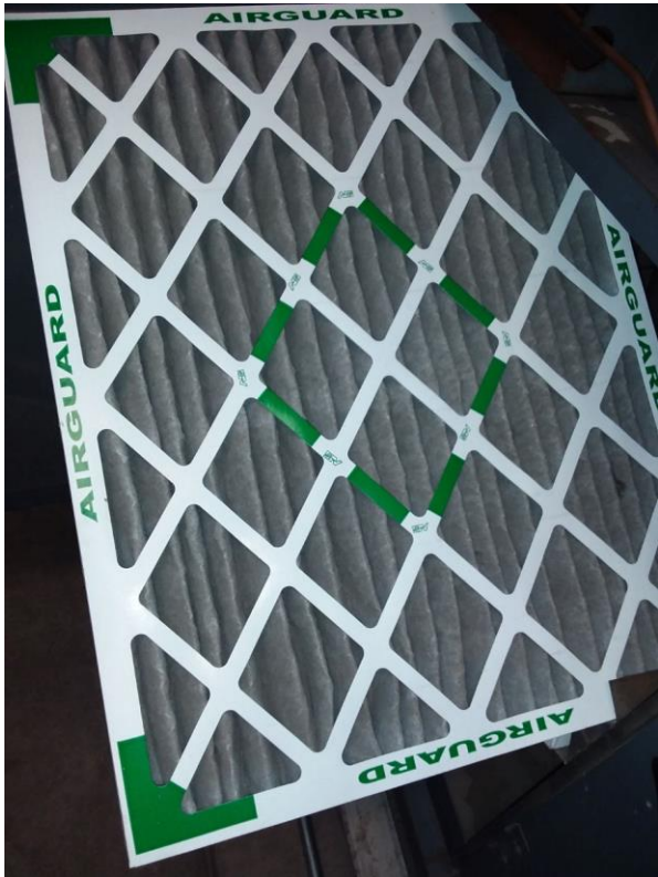
AHU_02 Mixed Main Filter Cleanliness
