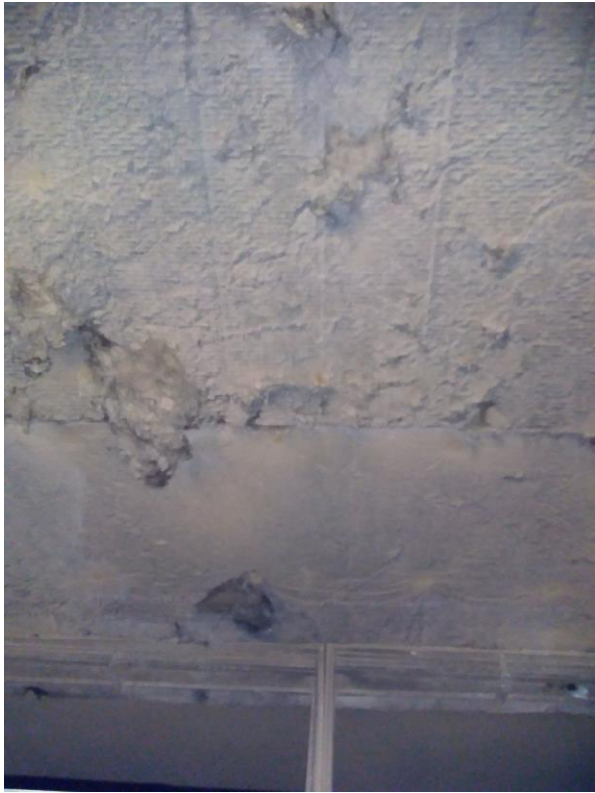
AHU_07 Interior Ducting
