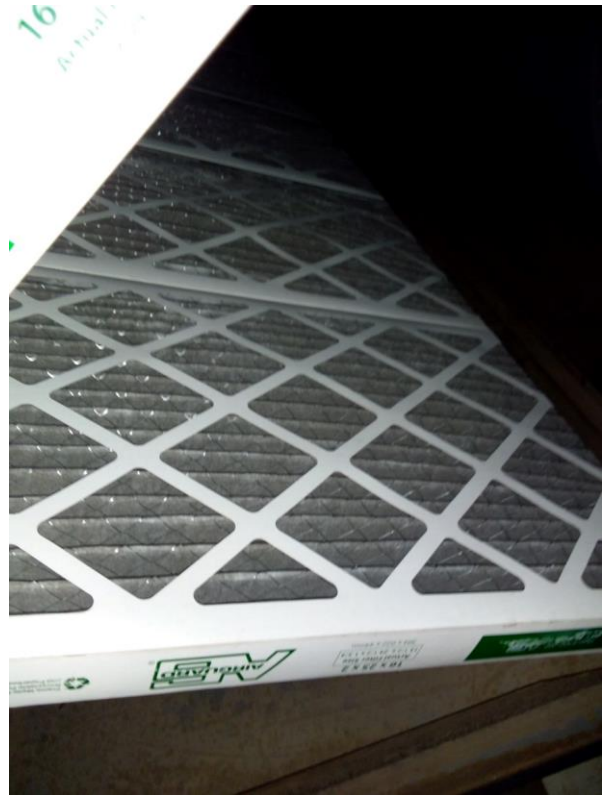
AHU_12 (100% RA) Return Main Filter Cleanliness
