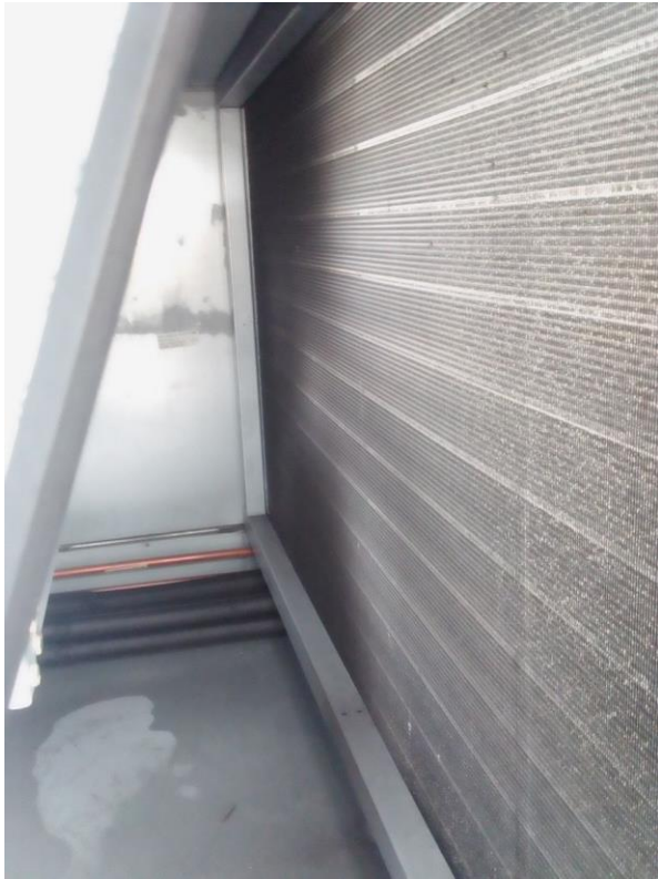
ERV-16 Heating Coils
