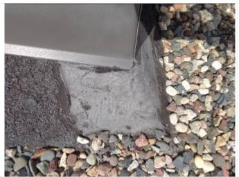
10. View of gray roof flashing material (404-GRF-A,B,C [POSITIVE]) present on each roof level.
