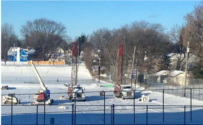
Drilling of geothermal wells at Johnson Senior High School in the baseball outfield.
