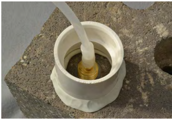
Figure 6. Water dam used for leak detection.
