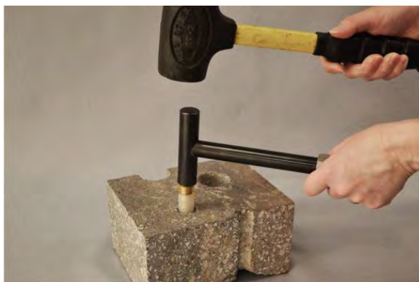
Figure 2. Installing the Vapor Pin™.
