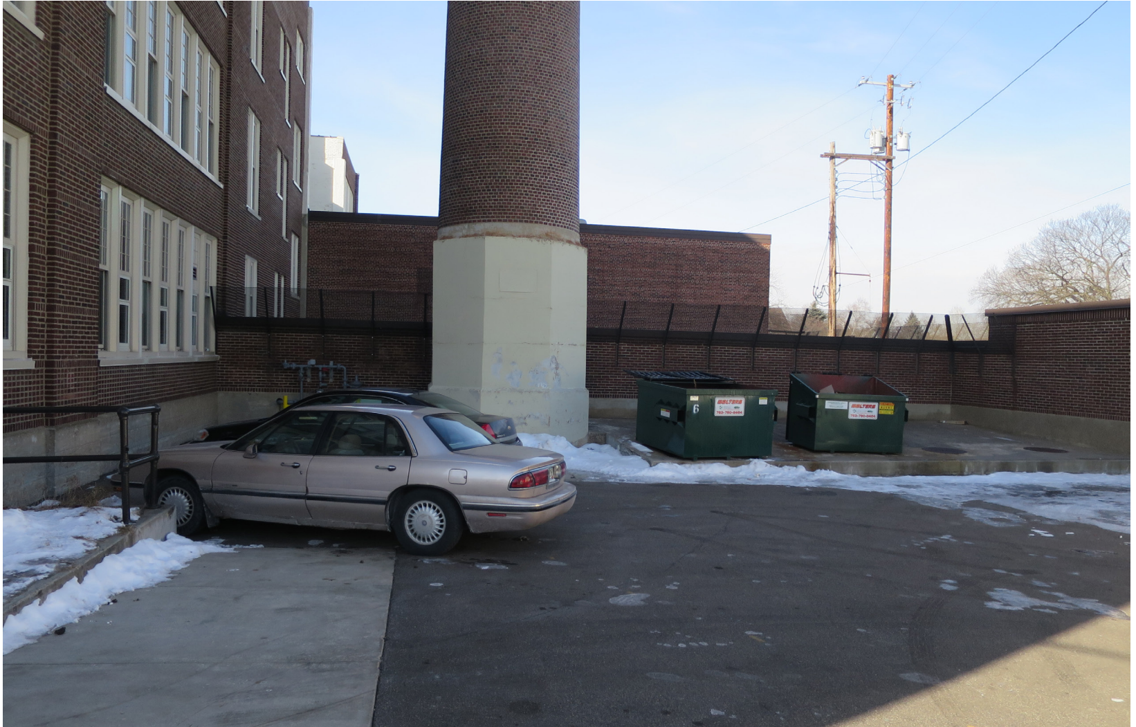
Existing Service Court
