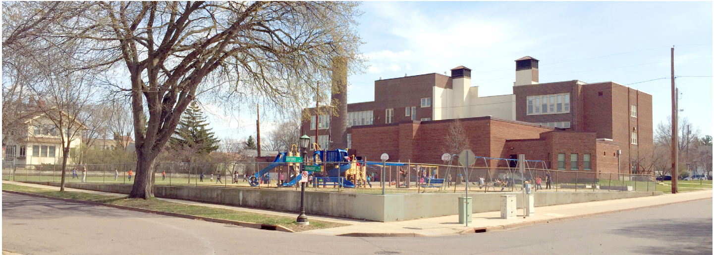
“Closed” Facade - Minimal or No Windows
