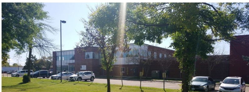
Photo of current north side of building; far left area will house addition
