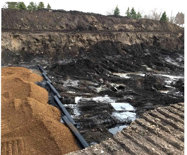
Images from top then left to right: Field during punchlist; center logo installed on field; track asphalt sheetflowing water; stormwater excavation prior to pumping water; excavation being filled with structural soil and geogrid; excavation being filled with structural soil and geogrid
