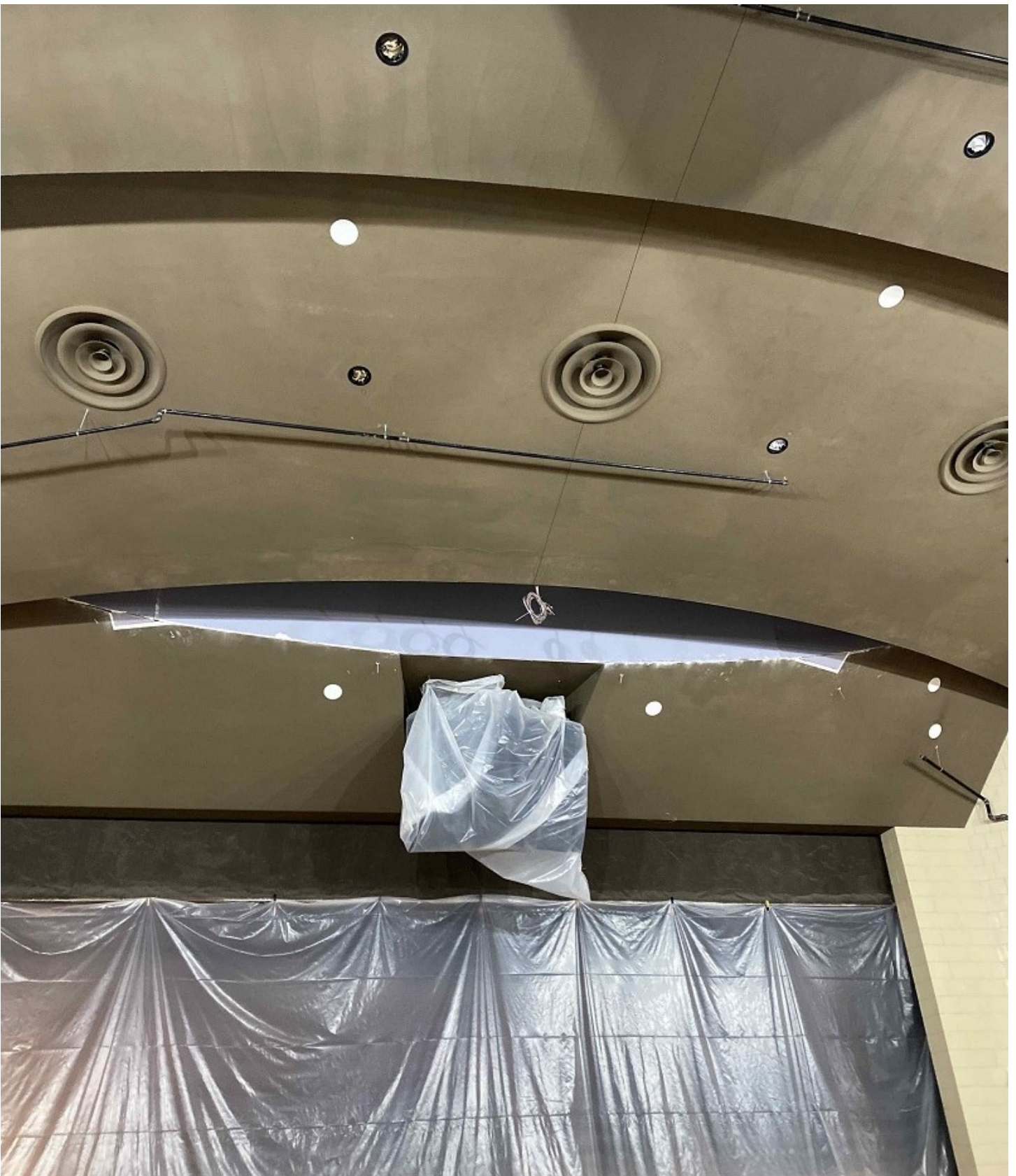
"Wing" wall above the ceiling to hide the equipment from the seating area site lines. (April 2021)
