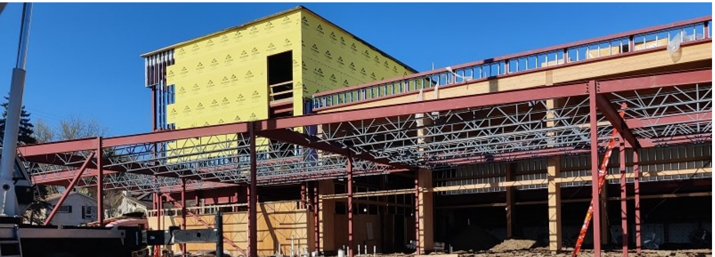
From top then left to right: Exterior sheathing in progress on three-story addition; ramp from main level to gym being prepped for concrete floor; first floor prepped for pouring concrete in three-story classroom addition; mechanical and electrical rough-ins, and interior wall framing being completed; steel framing, metal roof trusses and decking being completed on administration addition (April 2021)
