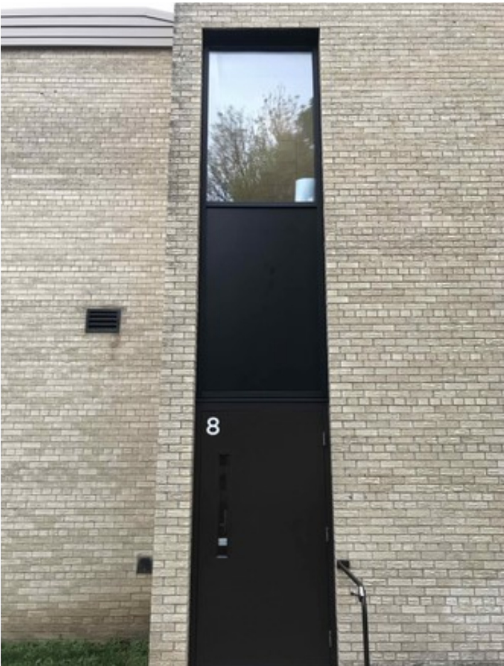
From left to right: St. Paul Music Academy – completed windows with new vent panel and insulated panel; completed windows; new panel and window above door; window from the interior (July 2021)
