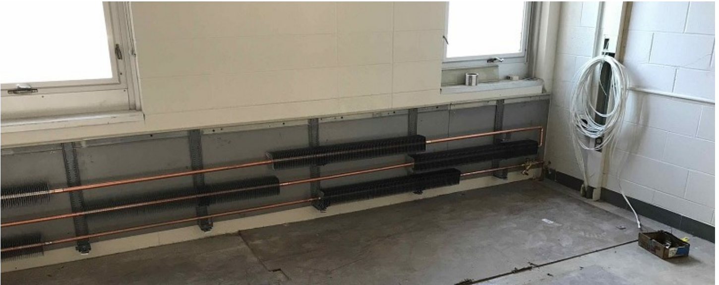
Top to bottom: New soffits along the walls in the classroom nearly ready to paint; new air handlers; new wall mounted fin tube radiation long the outside walls (July 2021)
