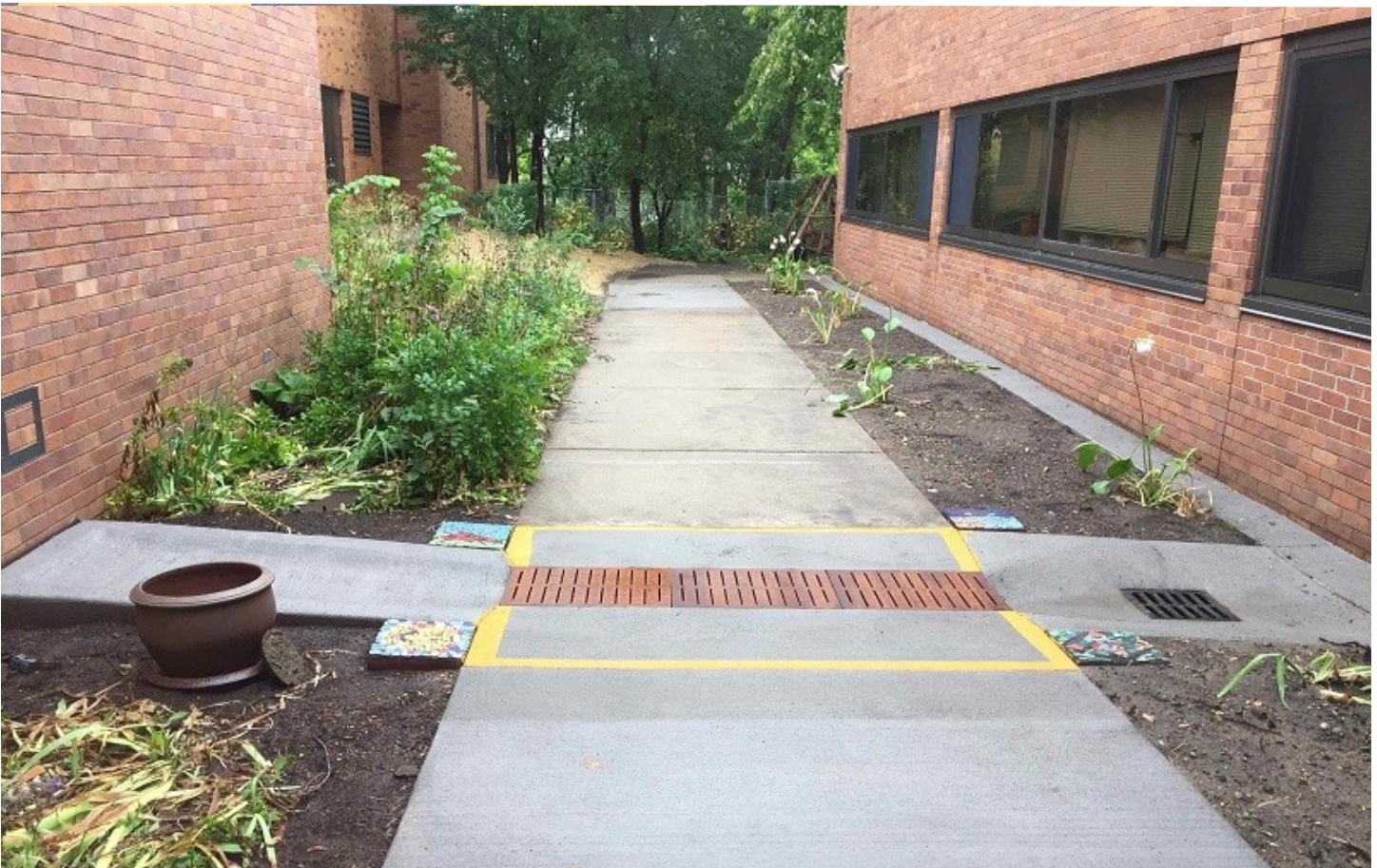
From top to bottom: Piping installed below existing floor; stormwater outlet ready for next summer; wheelchair accessible path across stormwater drainage (August 2021)
