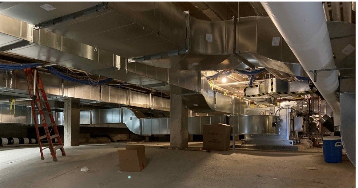
Top to bottom: New LED lighting, water sprinklers and ceiling tile; new ductwork and air handlers providing fresh air throughout the building (September 2021)
