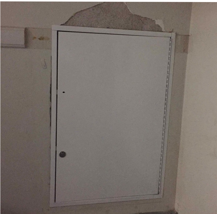
Photos from LEAP: Access panels for plumbing chases installed; patching and painting of adjacent wall in progress (November 2021)
