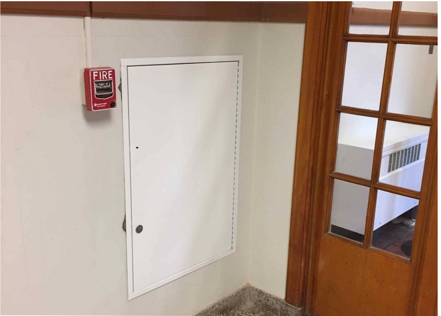
Photos from LEAP: Access panels for plumbing chases installed; patching and painting of adjacent wall in progress (November 2021)
