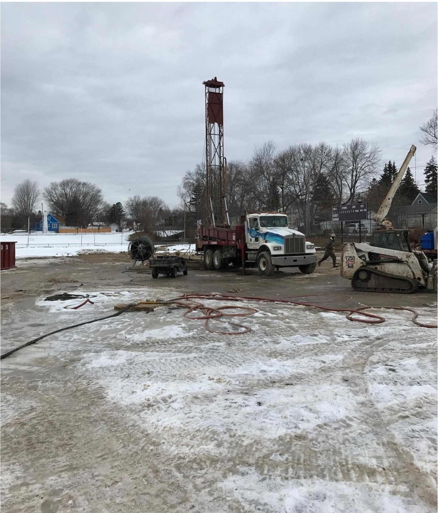
Geo-thermal vertical well drilling (March 2022)
