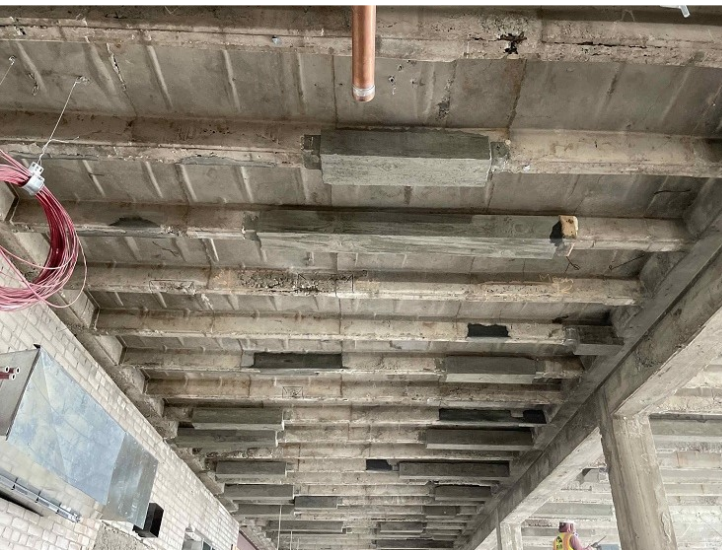
From left to right: Stone base around Circle Space nearing completion; demolition of old kitchen area; footings being set for new kitchen; drywall nearing completion for inclusive restrooms and changing rooms; concrete beam patching; mechanical rough-ins continue in fourth-floor corridor (March 2022)
