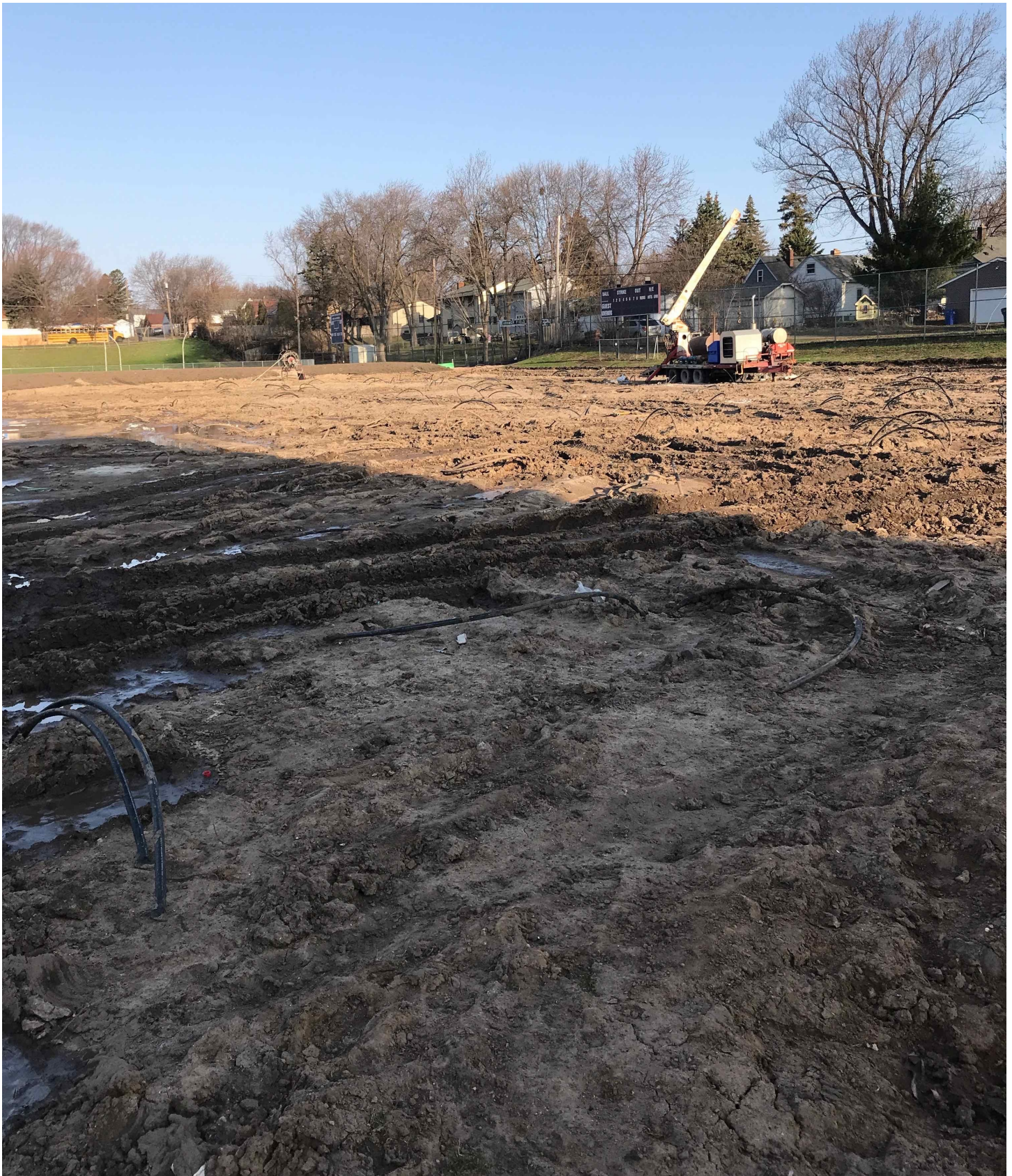
Geo-thermal vertical well drilling now complete (April 2022)
