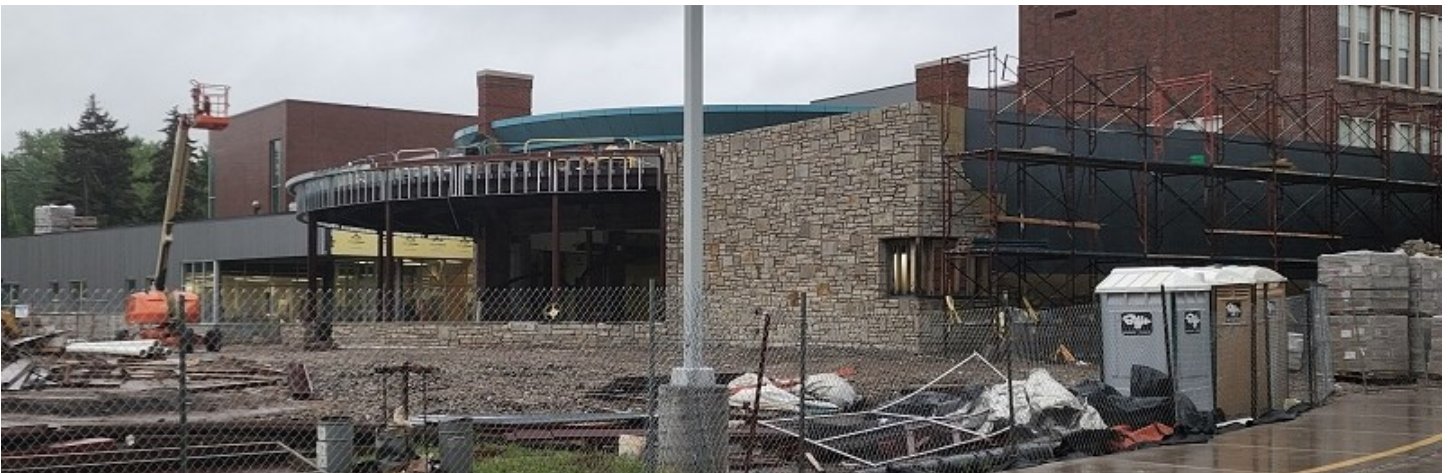
From left to right: Tiling of inclusive restroom; steel roof framing of kitchen addition; exterior steel wall framing of Circle Space; stone veneer for exterior of kitchen addition (May 2022)
