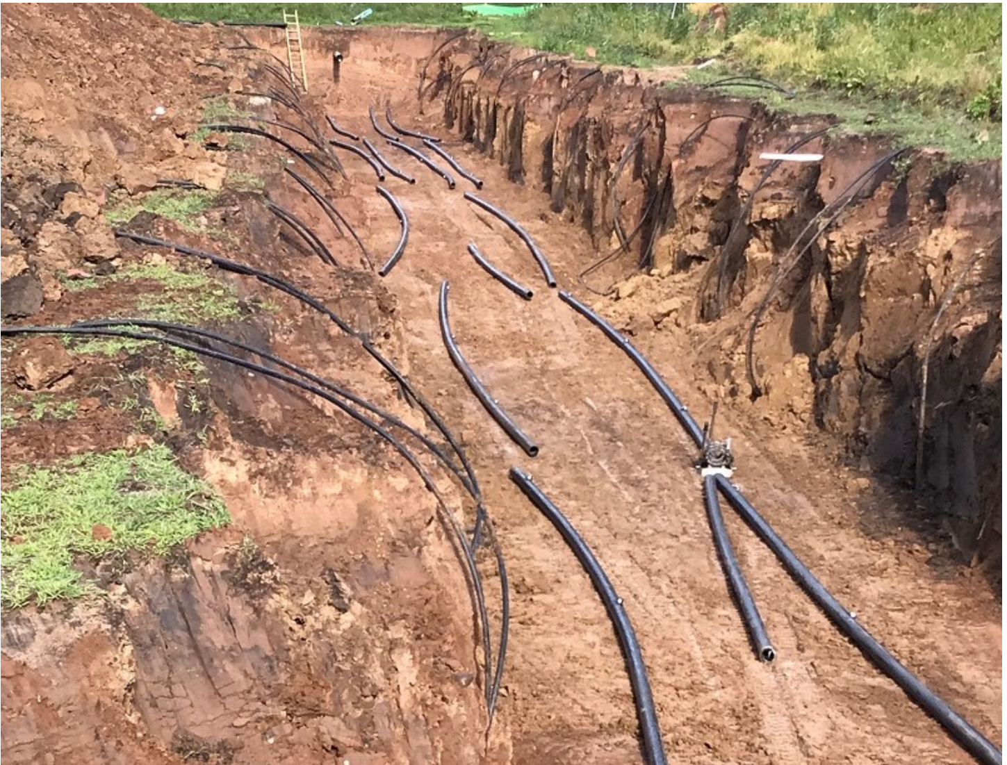
From top: Installation of new air ductwork; geo-thermal piping being connected and prepared for use (June 2022)
