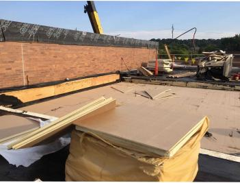
From top: Existing access hatch infilled; new access door opening has been cut; tapered insulation being installed in layers (August 2022)
