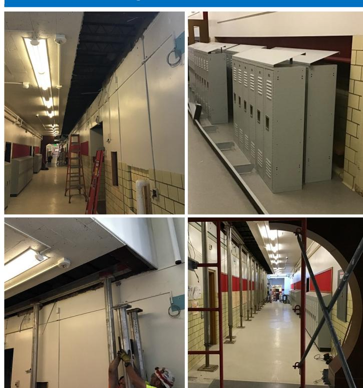
From top: Strip of ceiling in main corridor abated to facilitate installation of shoring and a temporary wall; lockers being temporarily relocated to make way for construction; shoring being installed to allow for planned wall demolition; main corridor facing east and soon to be divided by a temporary wall to separate students and staff from construction (July 2022)
