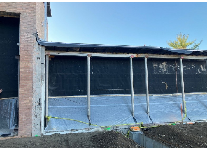
From top to bottom: Future loading dock and exterior wall foundations; concrete masonry unit (CMU) foundation walls will soon be below grade; moisture barrier and insulation on CMU foundation wall; shoring where the old stage and cafeteria were removed; footings and rebar for classroom addition and storm shelter (October 2022)
