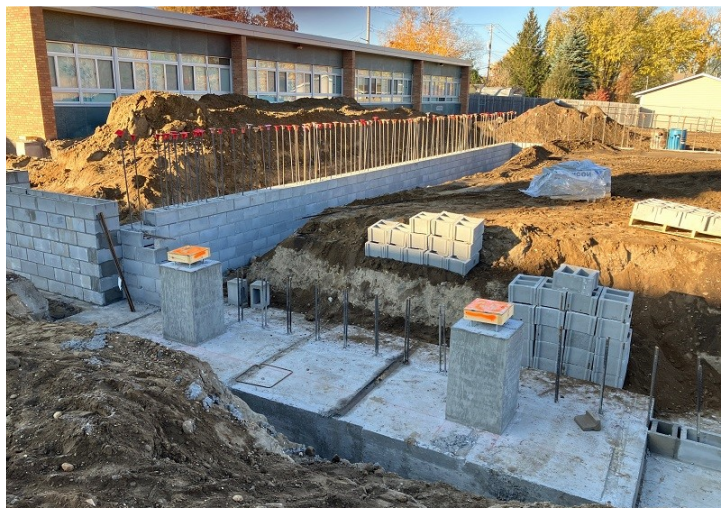
From top to bottom: Future loading dock and exterior wall foundations; concrete masonry unit (CMU) foundation walls will soon be below grade; moisture barrier and insulation on CMU foundation wall; shoring where the old stage and cafeteria were removed; footings and rebar for classroom addition and storm shelter (October 2022)
