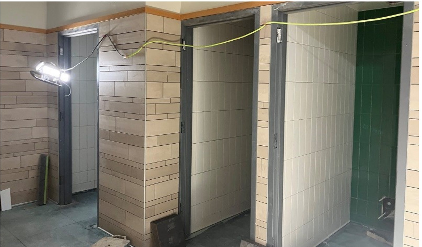
From top: Hallway renovation on third-floor; tile work in inclusive restroom (January 2023)
