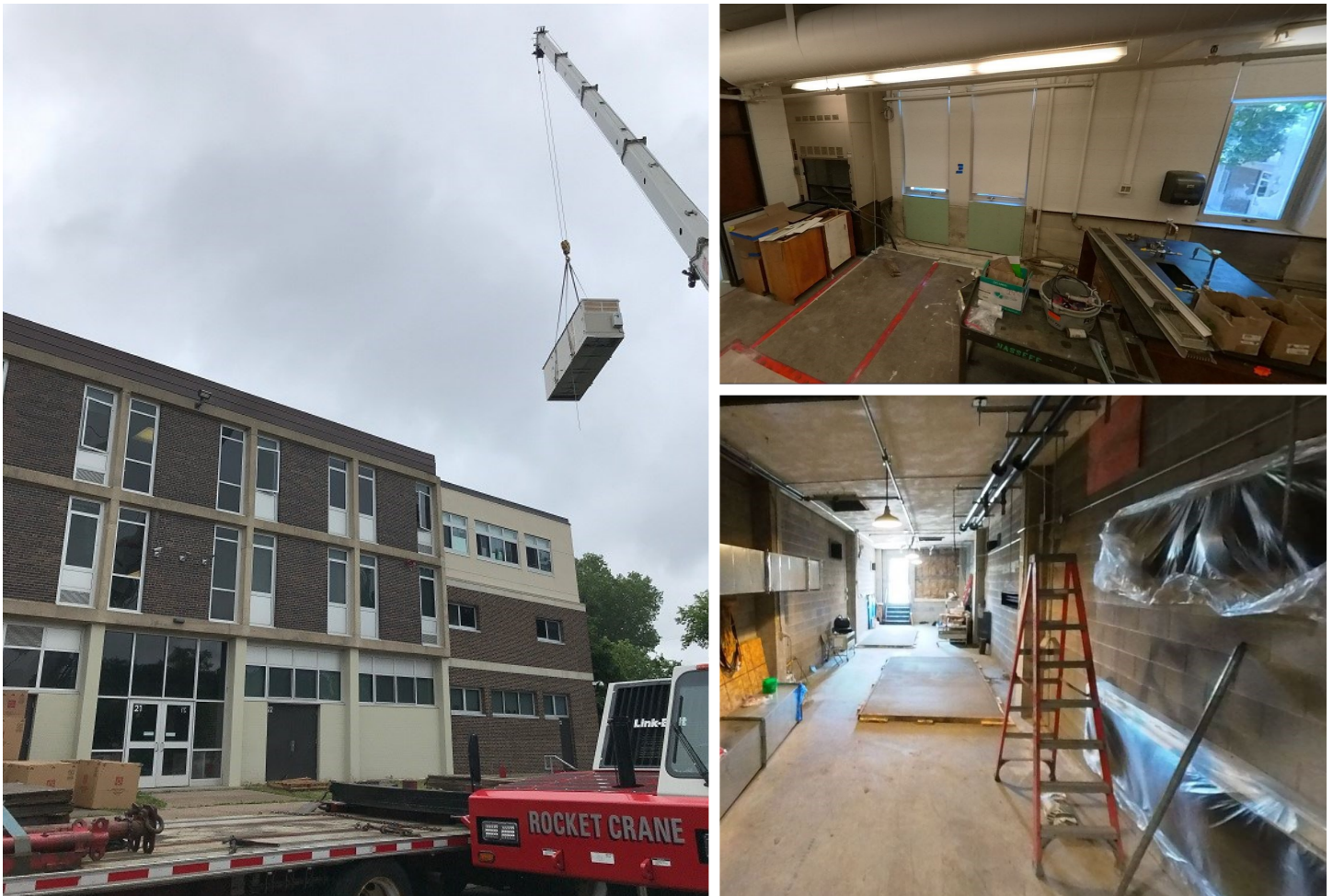
From top: New rooftop mechanical unit being lifted into place; old unit ventilators removed from classrooms; room prepped for new air handler units to provide improved air quality (June 2023)
