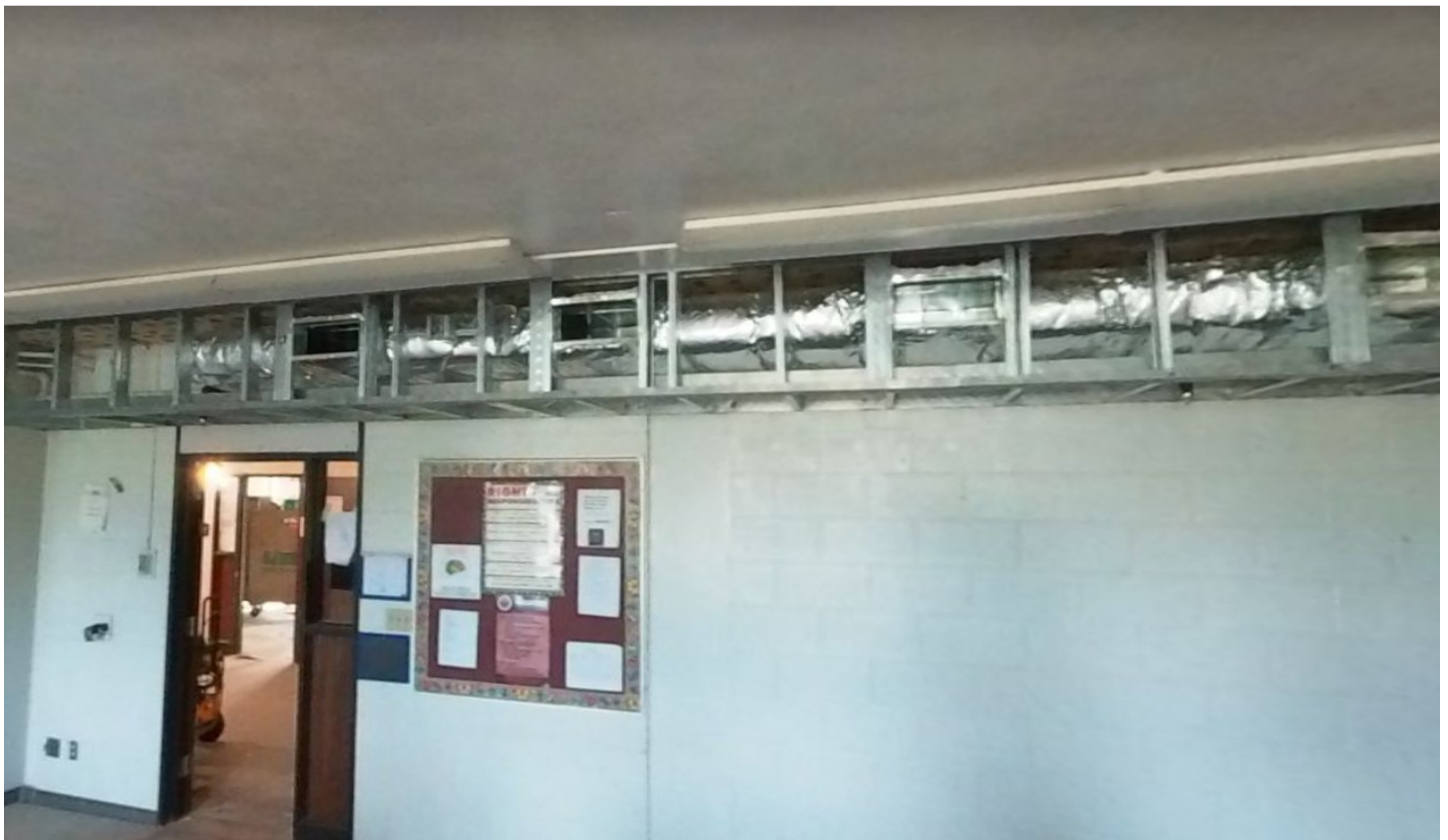
From top: Wall radiation being installed in classroom; drywall soffit that will house and hide new ductwork in classrooms (July 2023)
