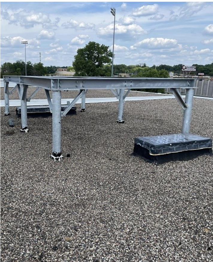
From top to bottom: Ductwork and hydronic installation; structural steel for new rooftop units; soffits housing ductwork and piping used in the majority of classrooms (July 2023)
