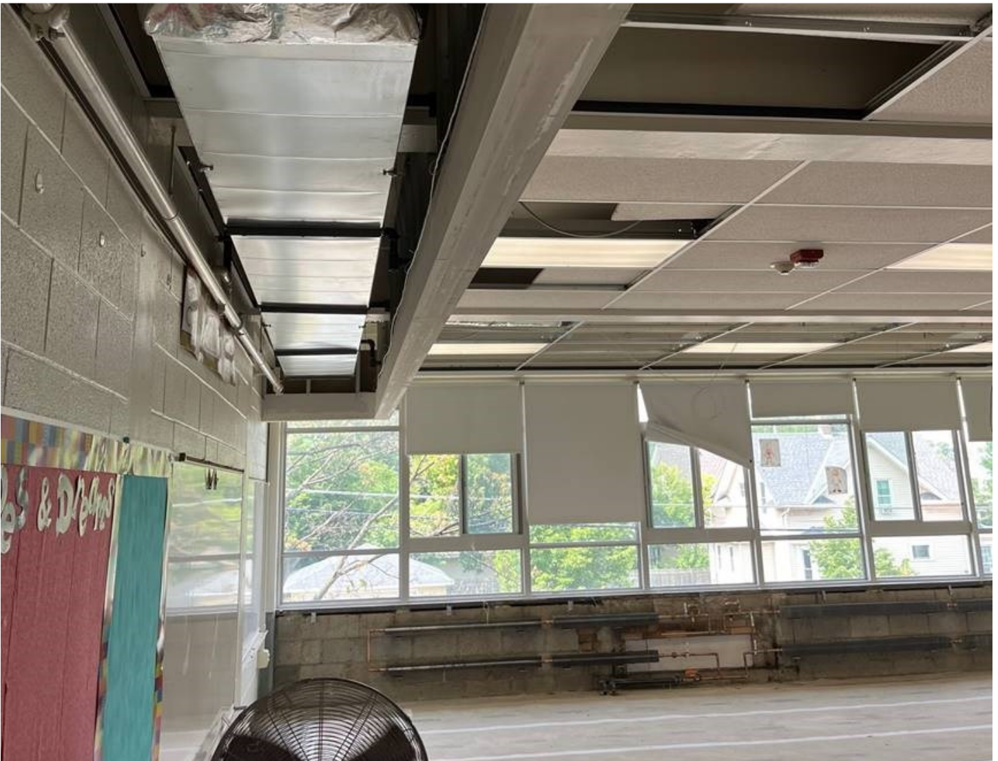
From top: New wall radiation in classroom being installed; new ductwork and soffits being installed in classroom (July 2023)
