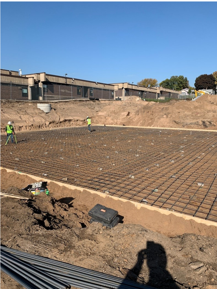
Top row: Buried utility lines; buried debris being removed; Bottom row: West underground storm water infiltration system being prepped and poured with concrete (October 2023)
