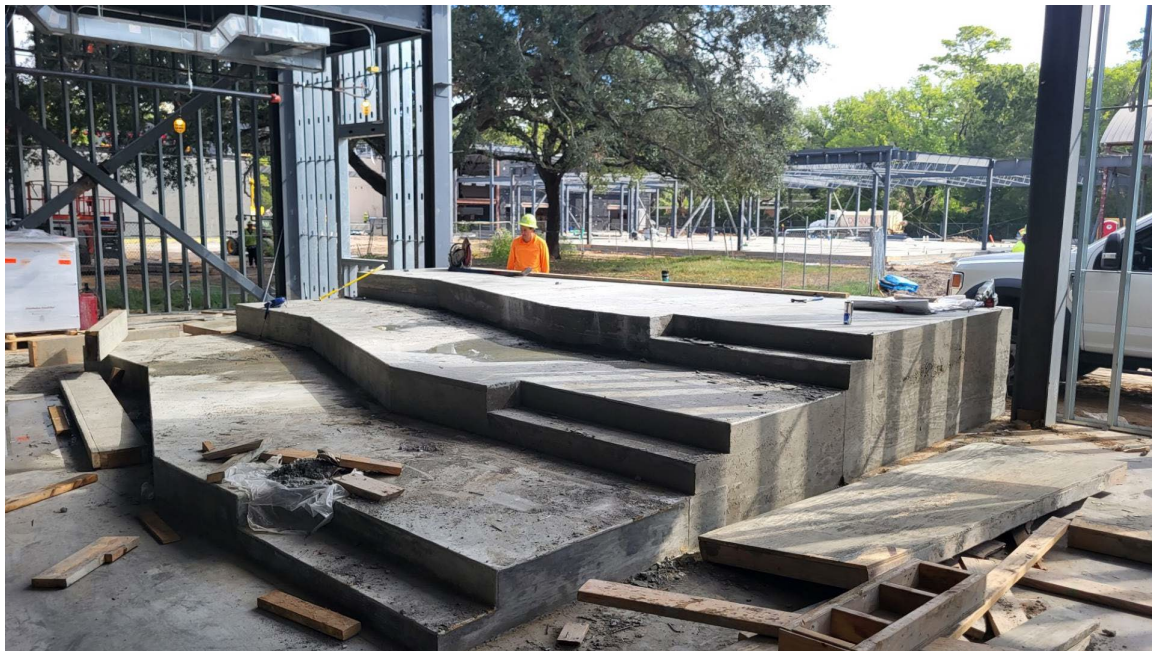
Area A Learning Stair concrete poured
