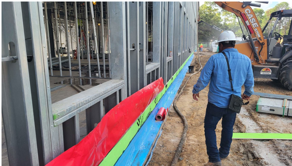
Area A Wall Base Flashing installation ongoing
