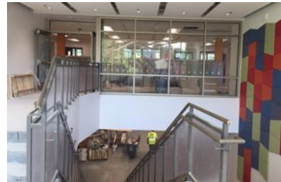
Main stairwell near front door (8/18)
