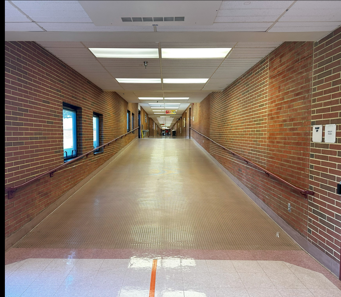
Existing ramp does not meet ADA accessibility
