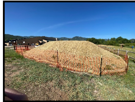
Completed main pile cap - west
