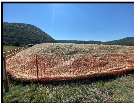
Completed cap and straw layer C&D Pile - east
