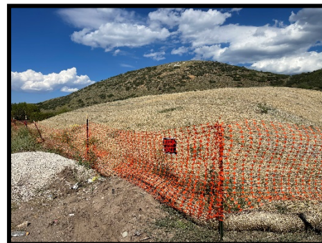
Posts, fencing, signage, erosion control.
