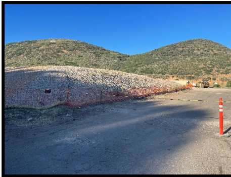
Completed main pile cap – northeast
