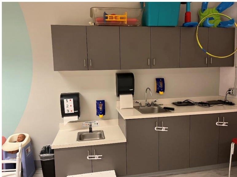
The faucet to the right, located in Room 114, was identified with lead levels above the action level of 15 \mu\text{g/L} .
