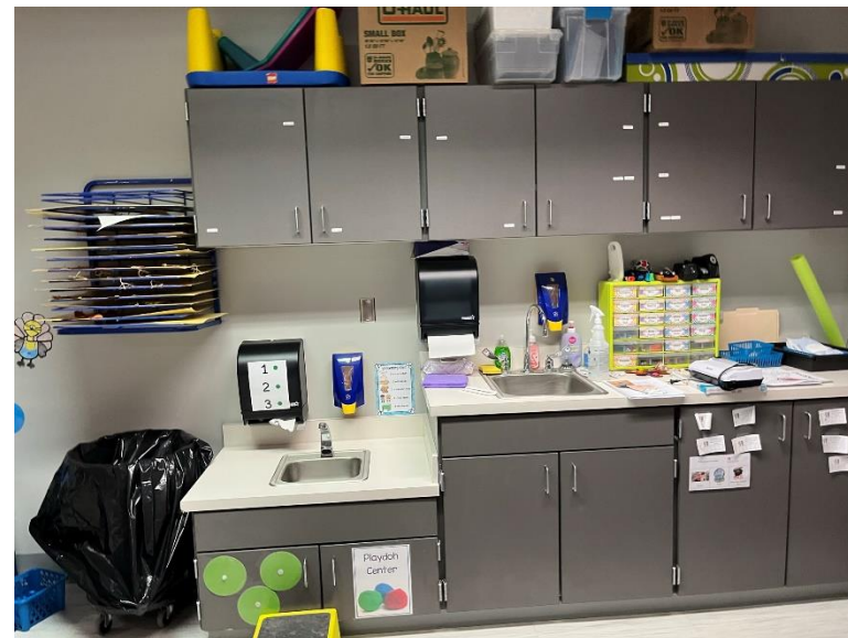
The faucet to the right, located in Room 112, was identified with lead levels above 5 \mu\text{g/L} .
