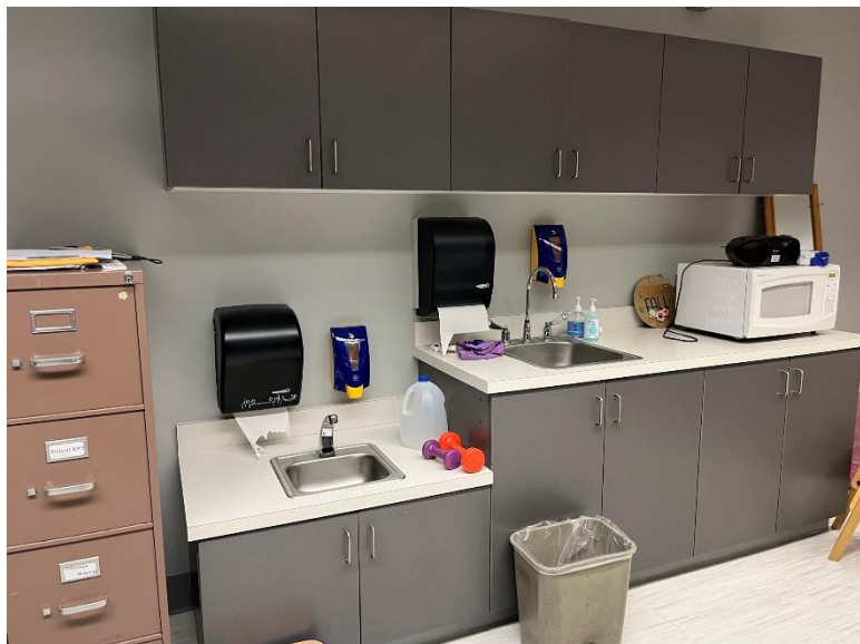
The right faucet located in Room 106 was identified with lead above the action level of 15 \mu\text{g/L} . The left fixture exceeded 5 \mu\text{g/L} .
