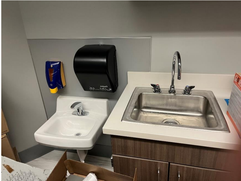
The fixture to the left, located in Room 102, was identified with lead levels above 5 \mu\text{g/L} and copper levels above 1,300 \mu\text{g/L} .
