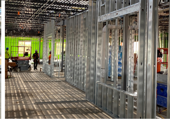
Interior Drywall Framing
