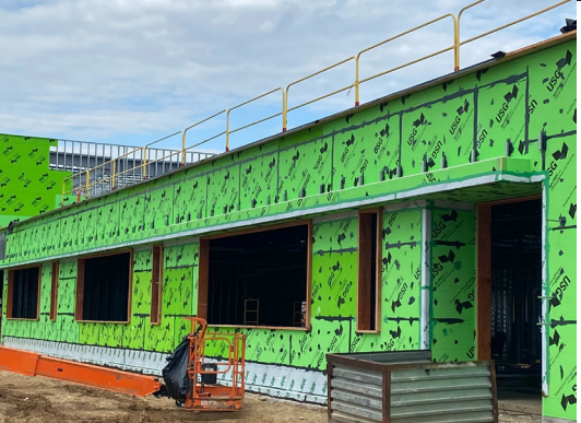
Exterior Framing and Sheathing
