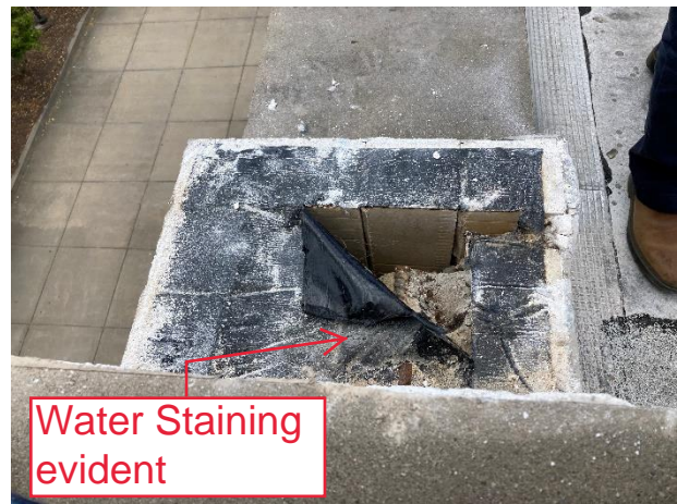
Self-Adhering waterproof underlayment does not extend to outside faces of wall.
