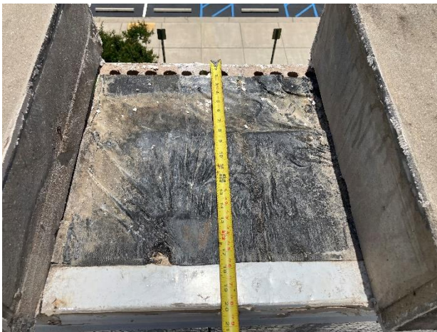
Trough and water staining evident.
