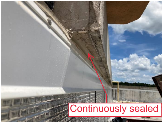
Interface of coping/parapet continuously sealed
