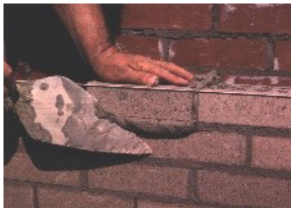
Photo 2 Cutting Excess Mortar
