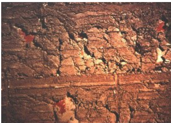
Photo 6 Poorly Filled Collar Joint
