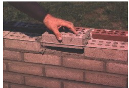
Photo 3 Placing the Closure
