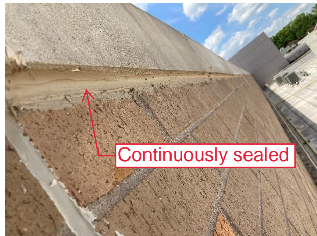
Interface of coping/parapet continuously sealed
