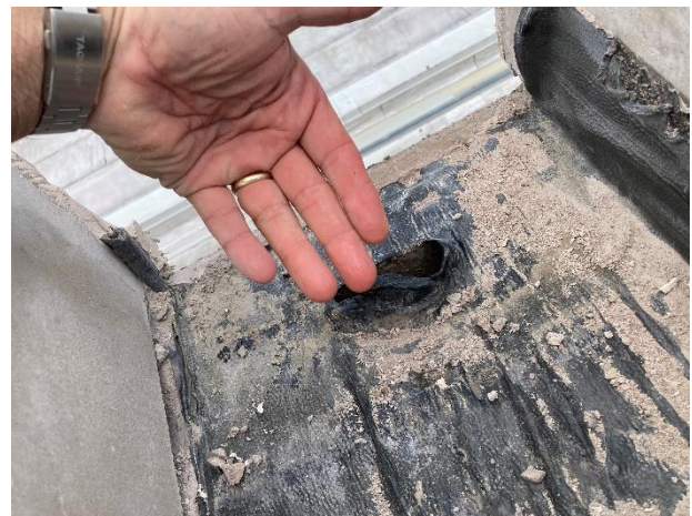
Underside of waterproof membrane wet
