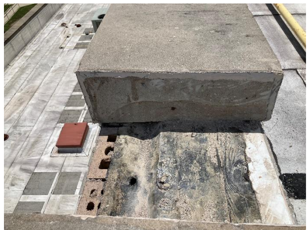
A trough exists in self-adhering waterproof underlayment.
