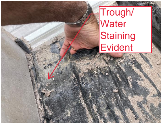
Underside of waterproof membrane wet
