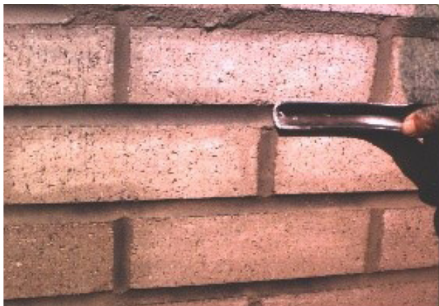
Photo 4 Concave Mortar Joints
