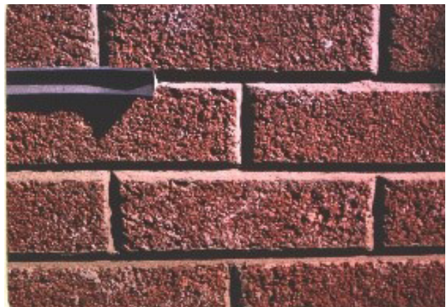
Photo 5 “V” Mortar Joints
