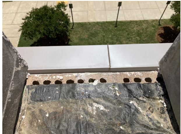
Brick mortar cells not covered.
