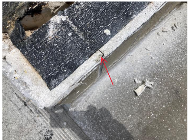
Water staining evident at crack in mortar joint
