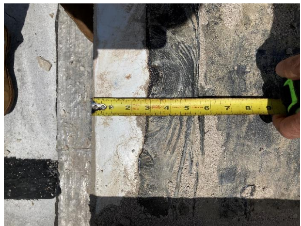
Self-Adhering waterproof underlayment stops approx. 3 inches from edge of wall.
