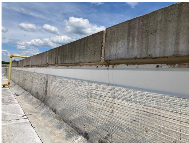
Interface of coping/parapet continuously sealed.
