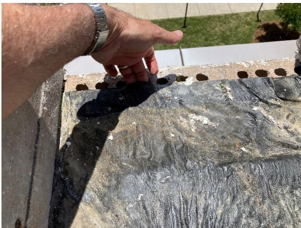
Self-Adhering waterproof underlayment does not extend to outside face of wall & not adhered.
