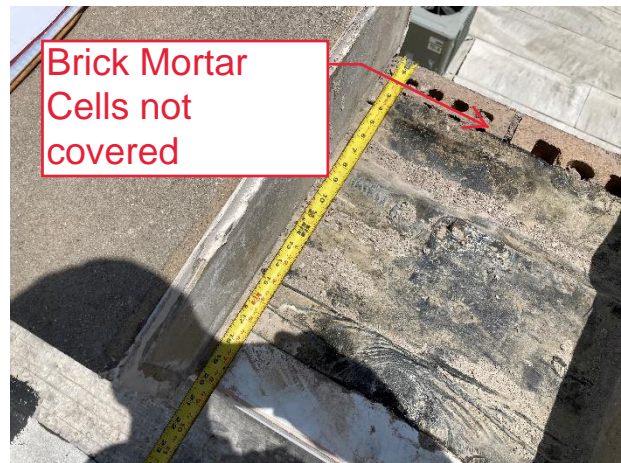
Self-Adhering waterproof underlayment does not extend to outside face of wall.
