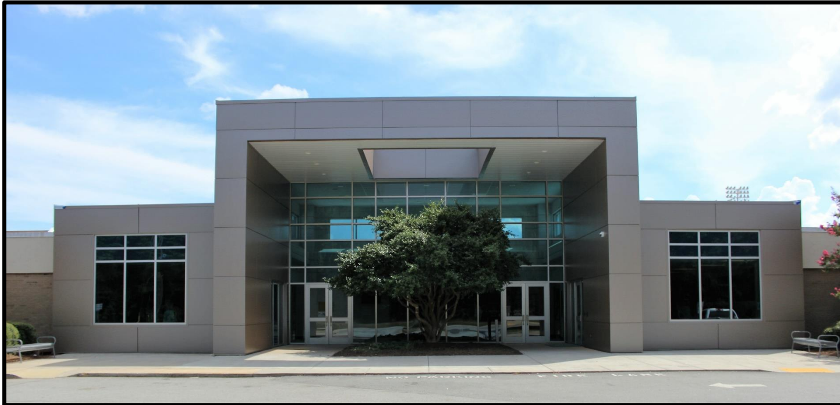
New Front Entrance
