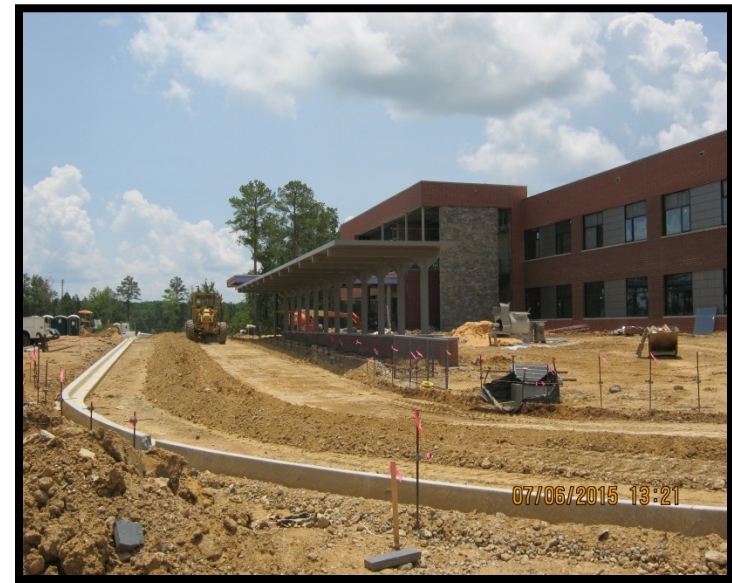
New Curb at Parent Drop-Off
