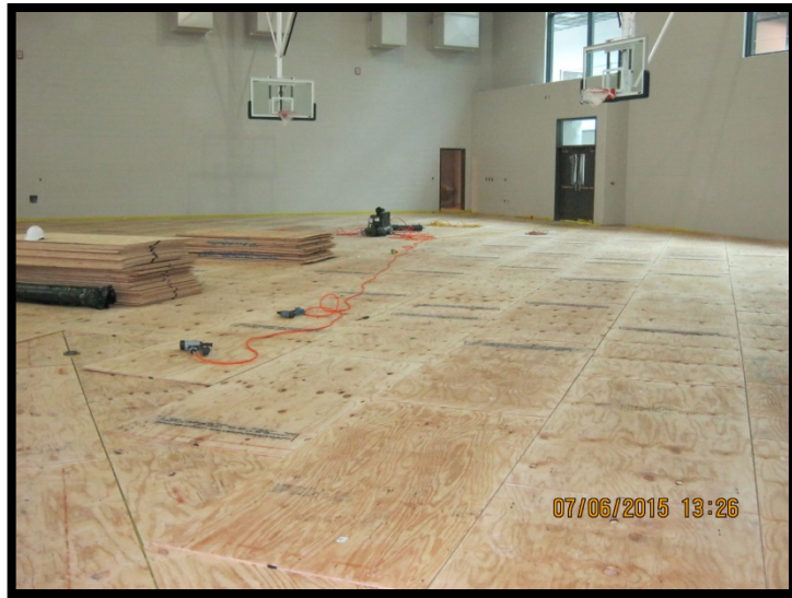
Gym Sub Floor
