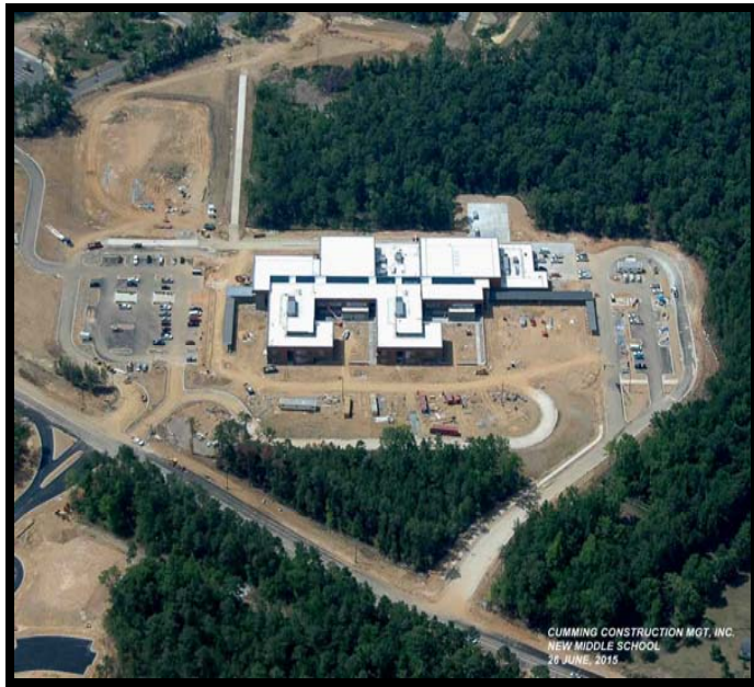
Front Aerial View
