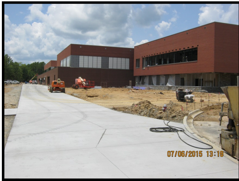
Concrete Drive Behind Building
