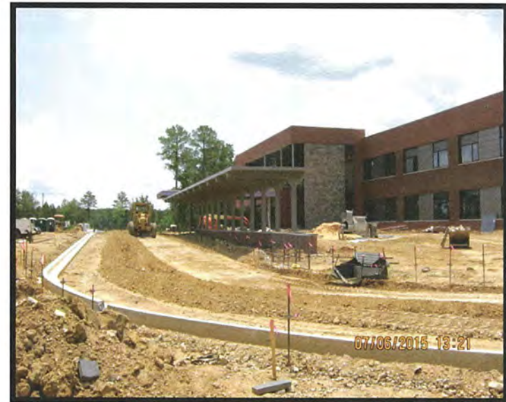
New Curb at Parent Drop-Off
