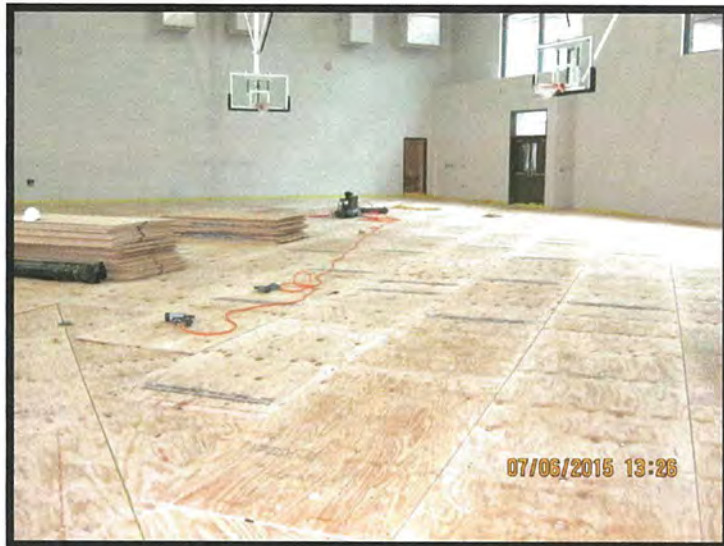
Gym Sub Floor
