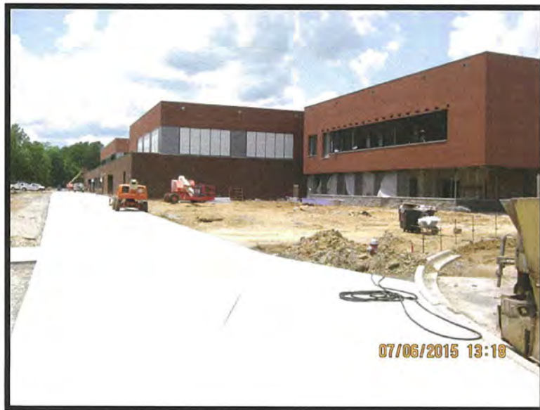
Concrete Drive Behind Building
