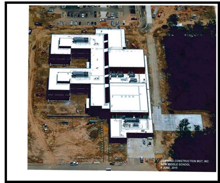
Side Aerial View from Loading Dock
