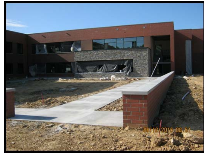
Stone Veneer in Courtyard
