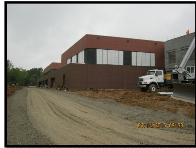
Rear Elevation At Gym
