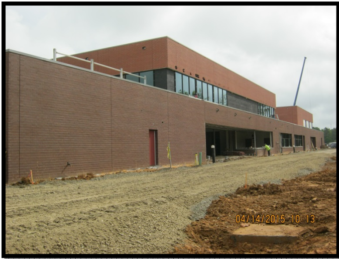
Rear Elevation Dining Room
