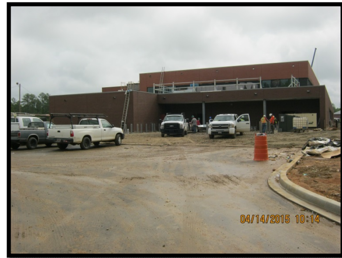
Entrance to Kitchen Loading Dock
