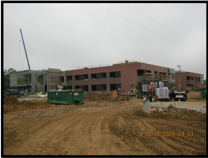
Entrance At Administrative & Classroom Wing
