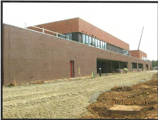
Rear Elevation Dining Room
