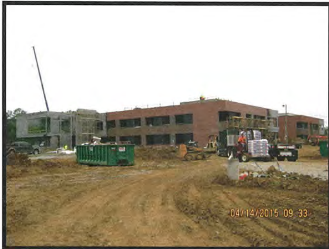
Entrance At Administrative & Classroom Wing
