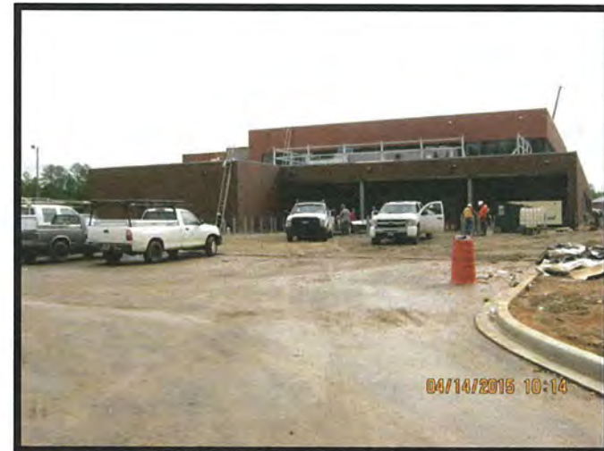
Entrance to Kitchen Loading Dock
