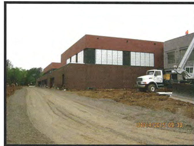
Rear Elevation At Gym
