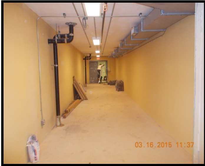
Interior Connector From Auditorium to Classroom Wing
