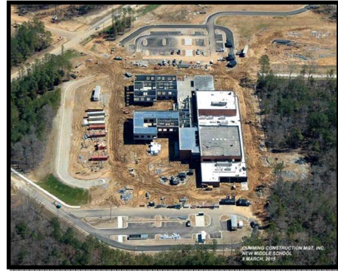
Overall View Chapin Middle School
