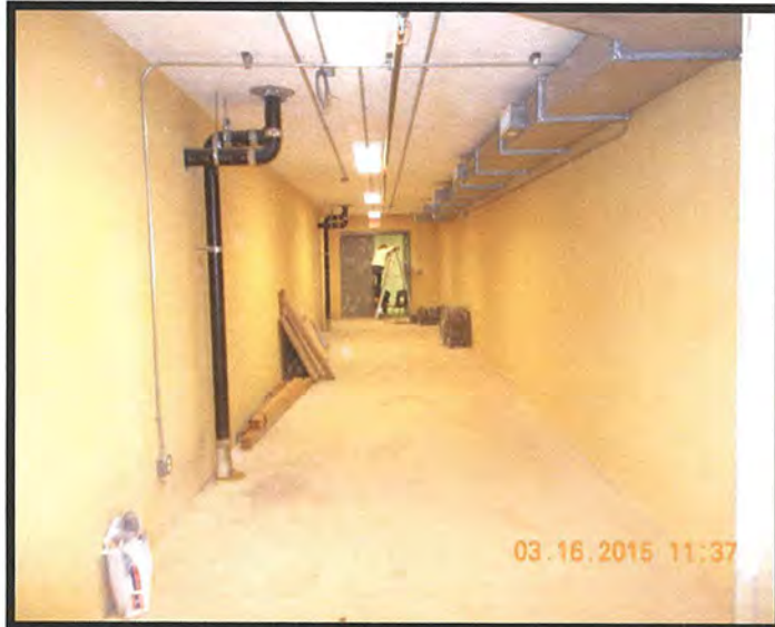
Interior Connector From Auditorium to Classroom Wing
