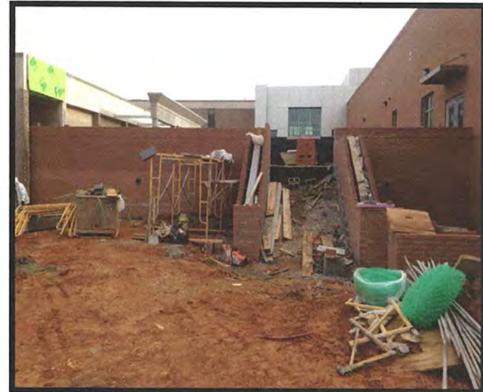
Exterior Amphitheater Entrance Way
