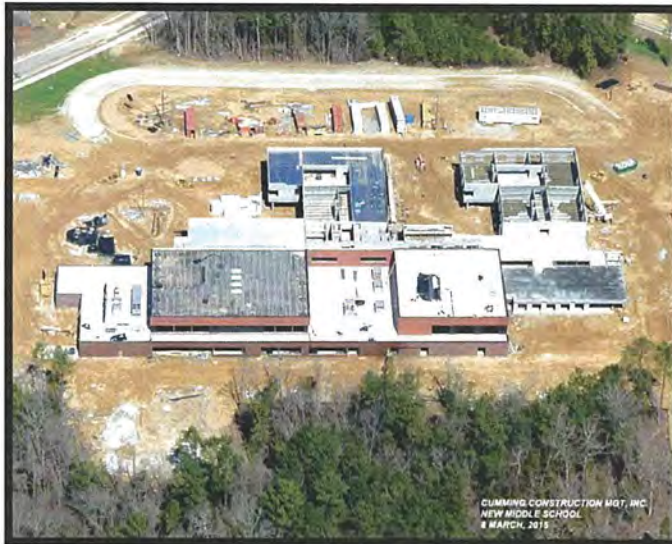
Rear View Chapin Middle School
