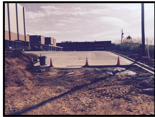
Loading Dock Concrete Pavement
