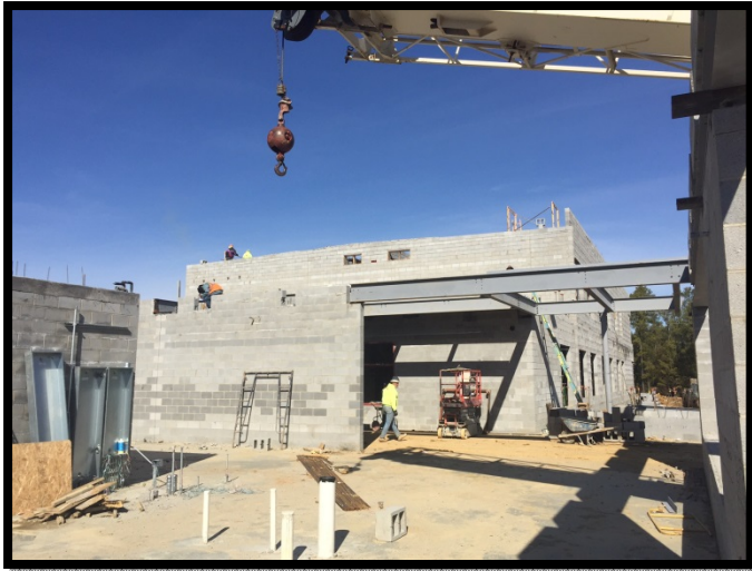
Structural Steel at Administration Area
