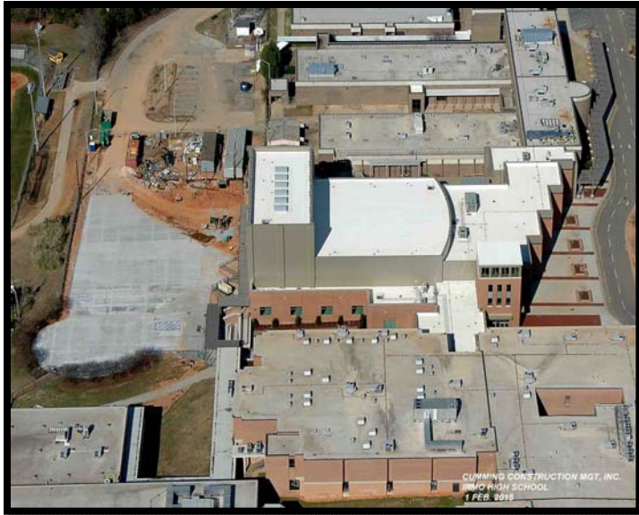
New Auditorium along St. Andrews
