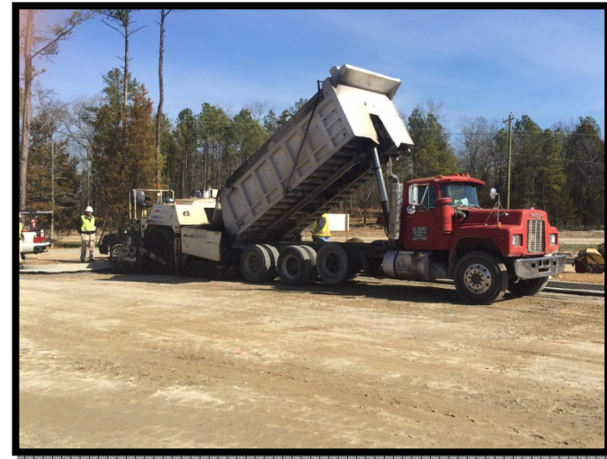
Parking Lot Asphalt Pavement
