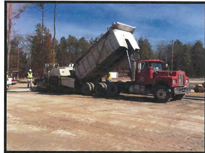
Parking Lot Asphalt Pavement
