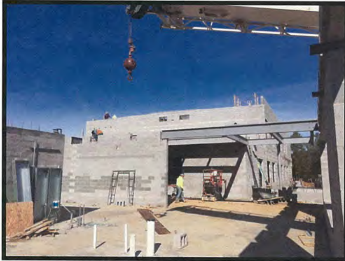
Structural Steel at Administration Area
