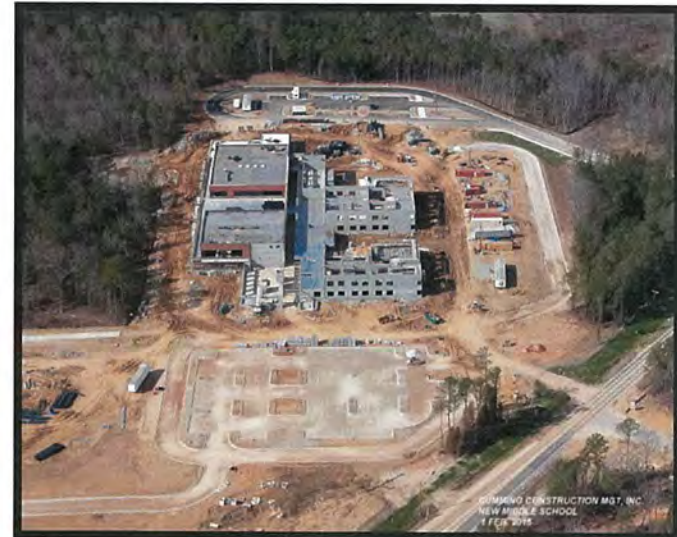
Chapin Middle School Site from Spring Hill High School
