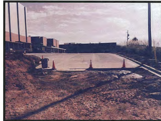
Loading Dock Concrete Pavement
