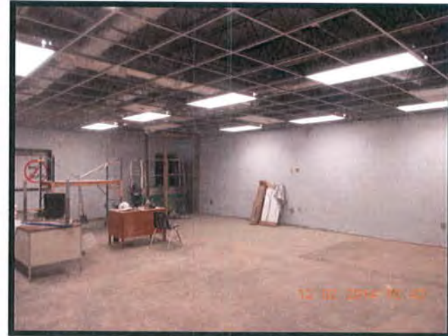
New Classroom Space
