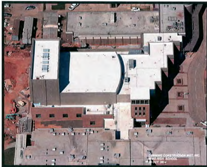
New Auditorium along St. Andrews
