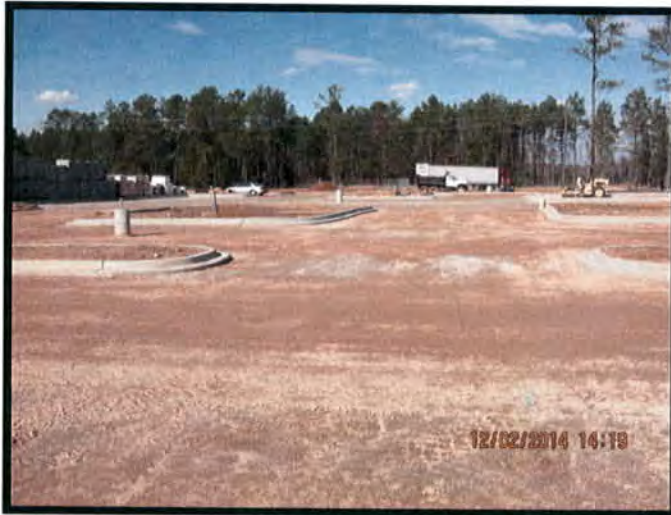
Grading / Curb and Gutter
