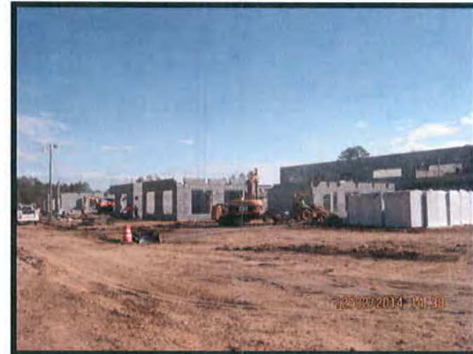
Classroom Wing Masonry
