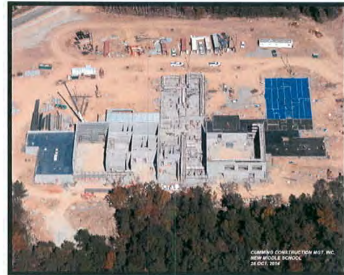
Slabs and Decking
