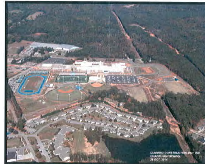
Site Aerial towards Columbia Avenue
