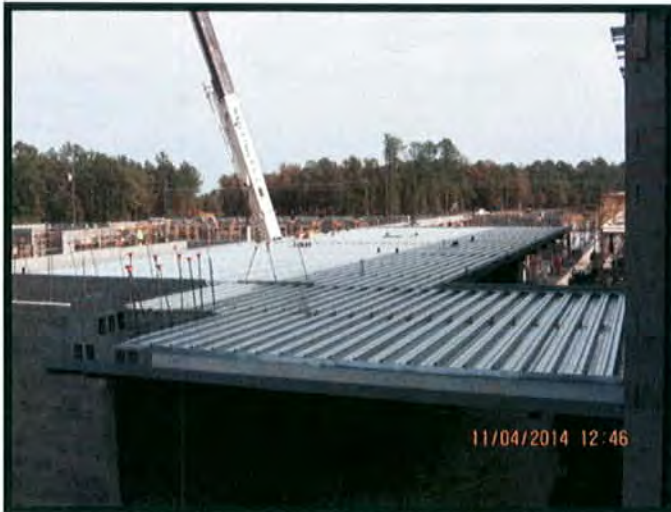
Second Level Decking
