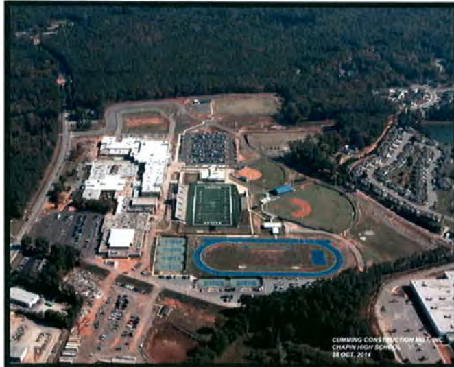
Site Aerial along Columbia Avenue
