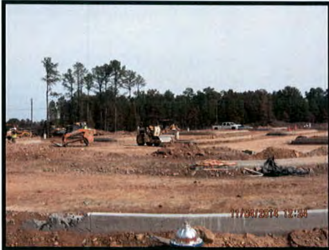
Grading / Curb and Gutter
