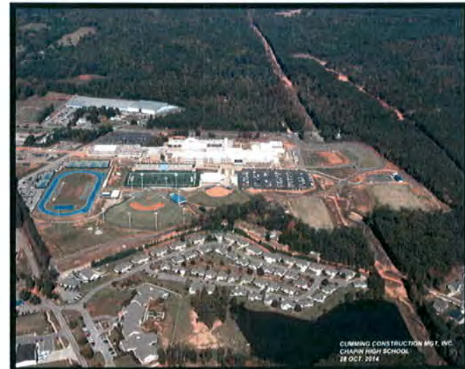
Site Aerial towards Columbia Avenue
