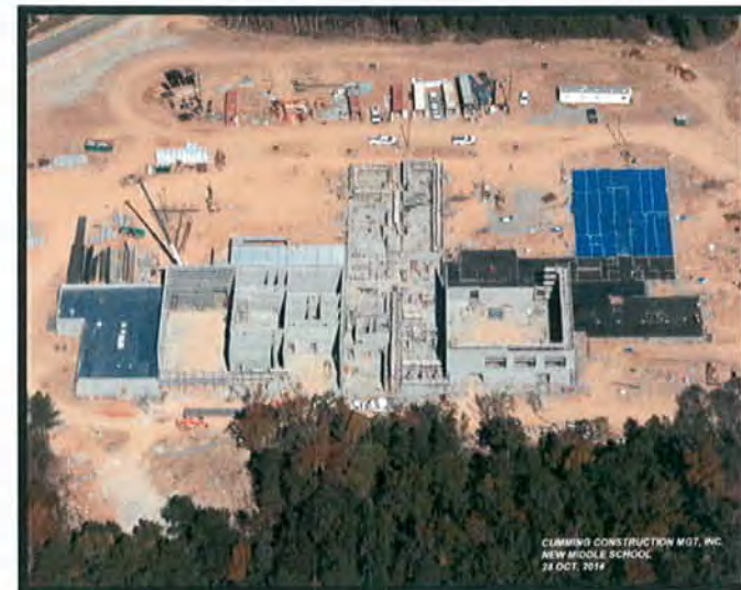
Slabs and Decking
