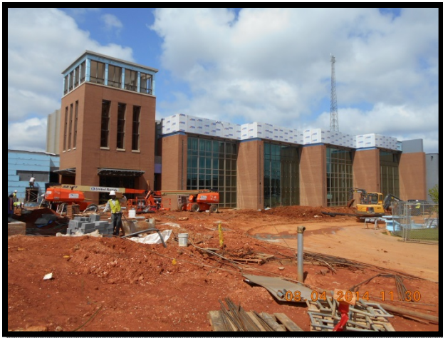
Front of New Auditorium
