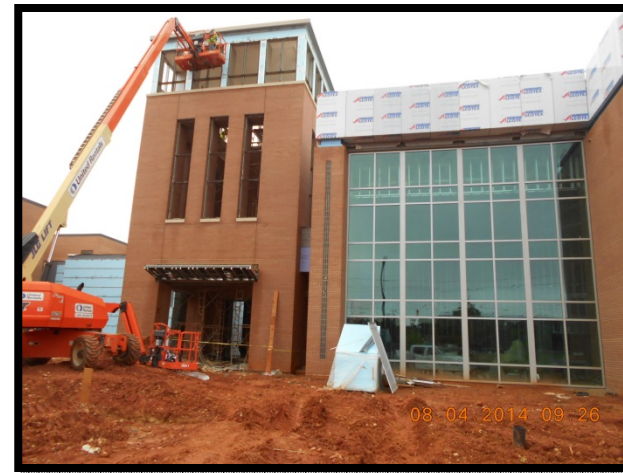
Front of New Auditorium
