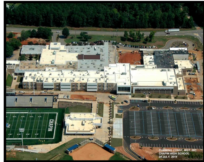
Site Aerial towards Columbia Avenue
