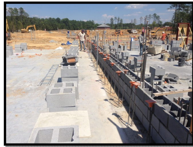
Masonry Being Installed
