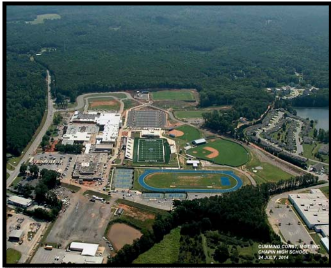
Site Aerial along Columbia Avenue
