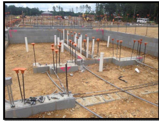
Foundations and Under Slab Rough In
