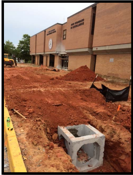
Existing Main Entrance
