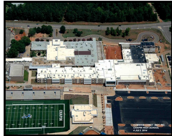
Site Aerial towards Columbia Avenue
