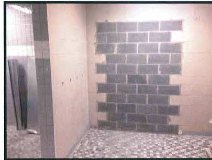
Masonry Infill
