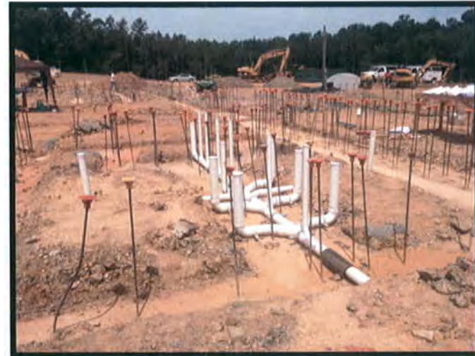
Footing Installation & Under Slab Rough In
