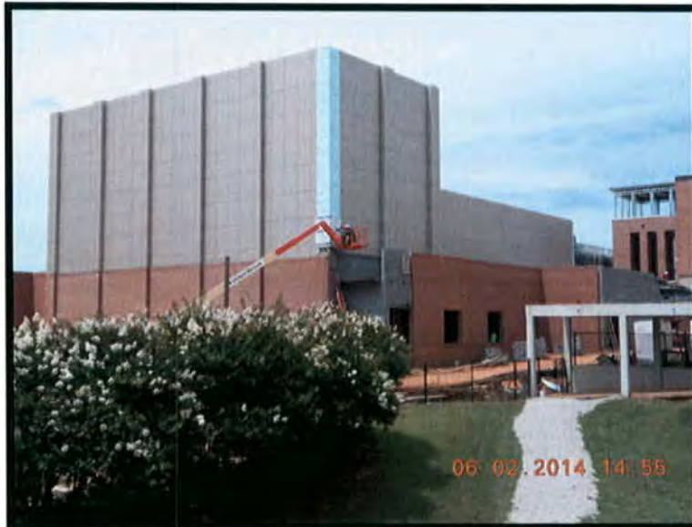
New Auditorium Metal Panels
