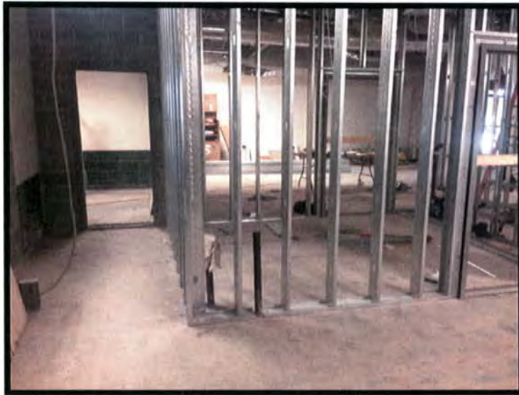
New Walls Being Installed
