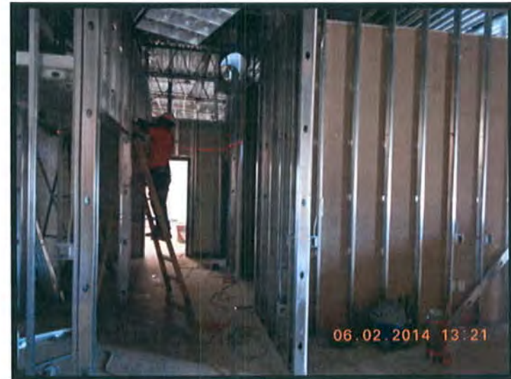
Renovation at CATE
