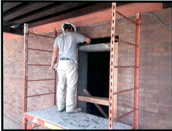
New Door Being Installed
