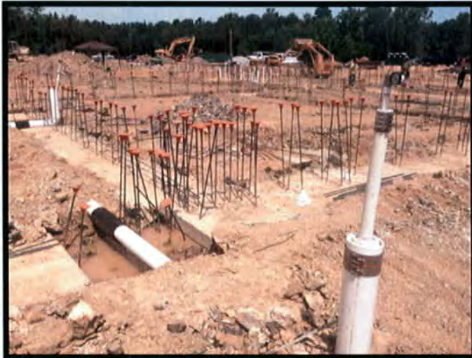
Footing Installation & Under Slab Rough In
