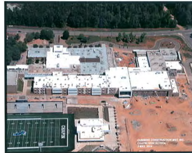
Site Aerial towards Columbia Avenue
