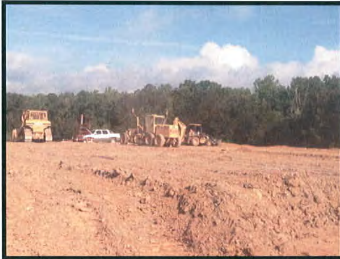
Soccer Field Grading
