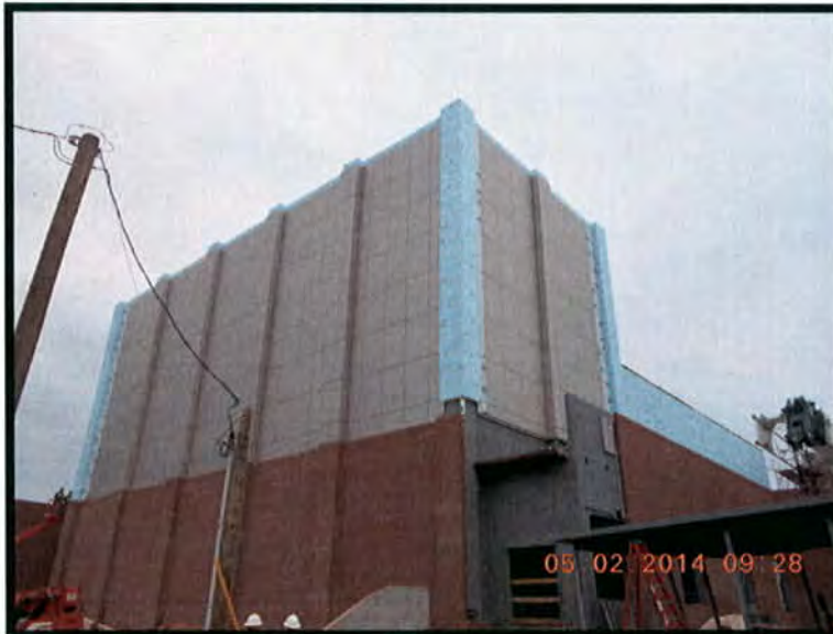
New Auditorium Metal Panels
