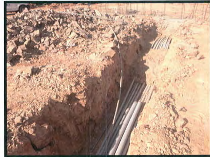
Electrical Rough In
