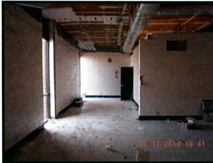
Renovation at CATE
