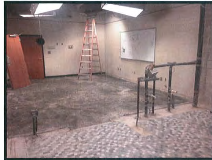
Existing Building Renovation
