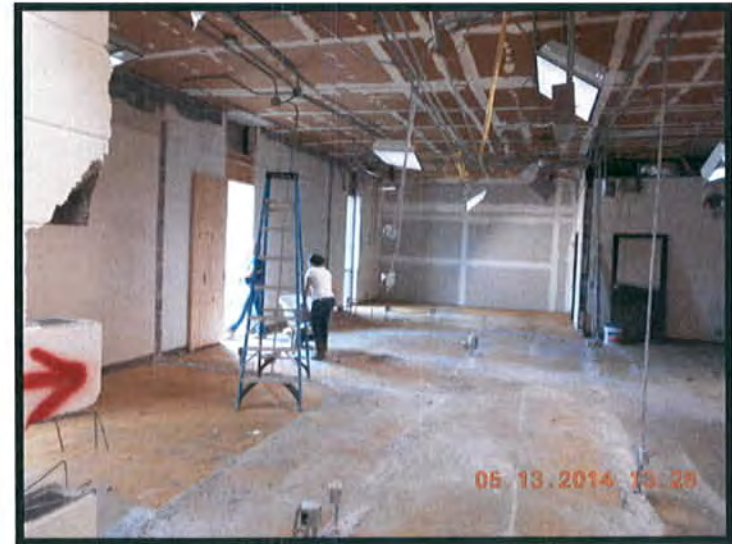
Renovation at CATE
