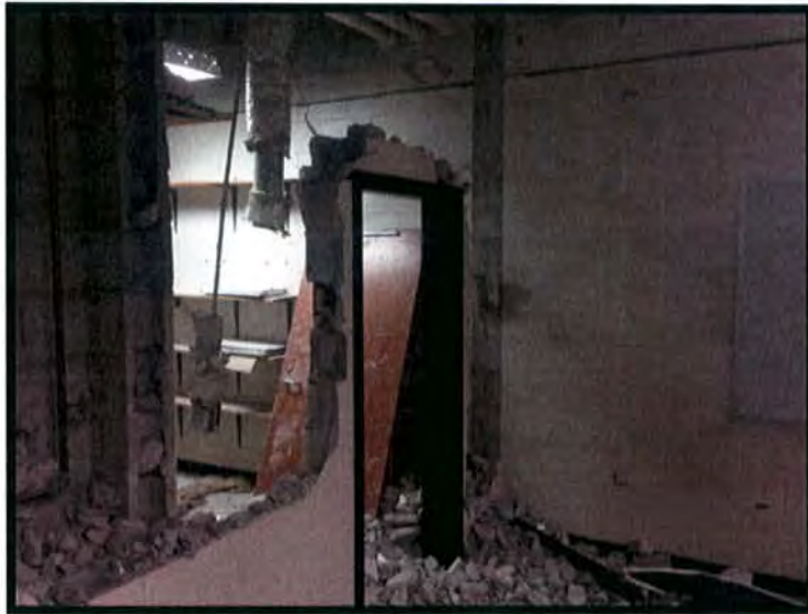
Existing Building Demo
