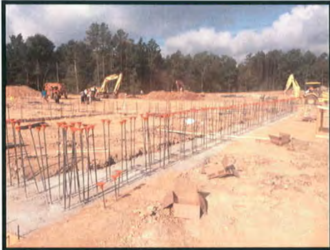
Footing Installation
