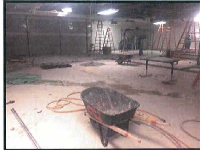
Existing Building Demo
