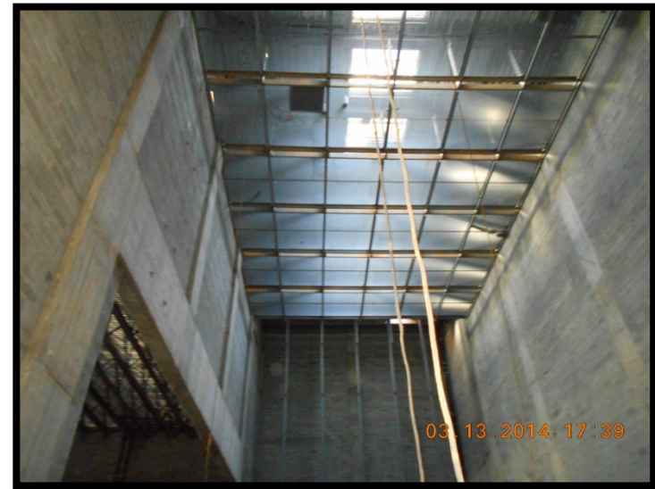
New Auditorium Stage Area
