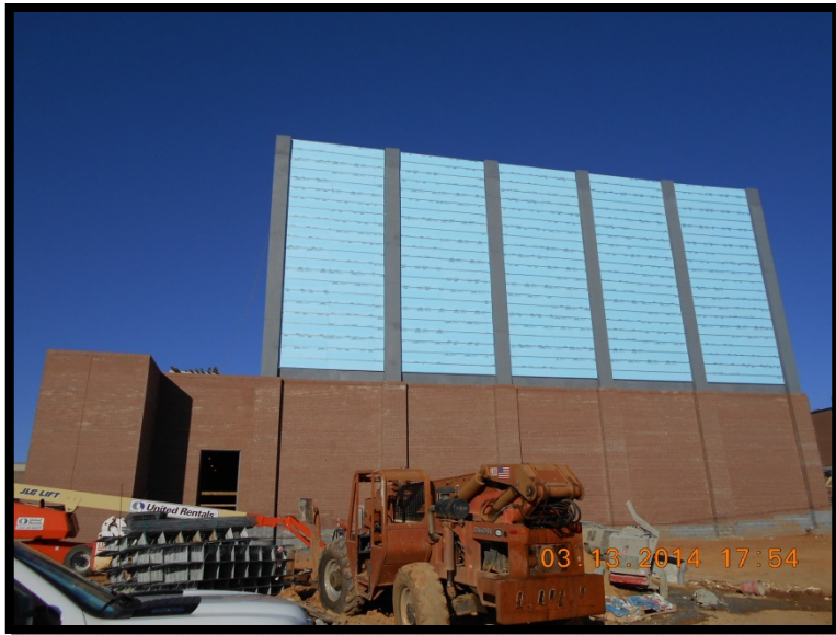
New Auditorium Brick Installation
