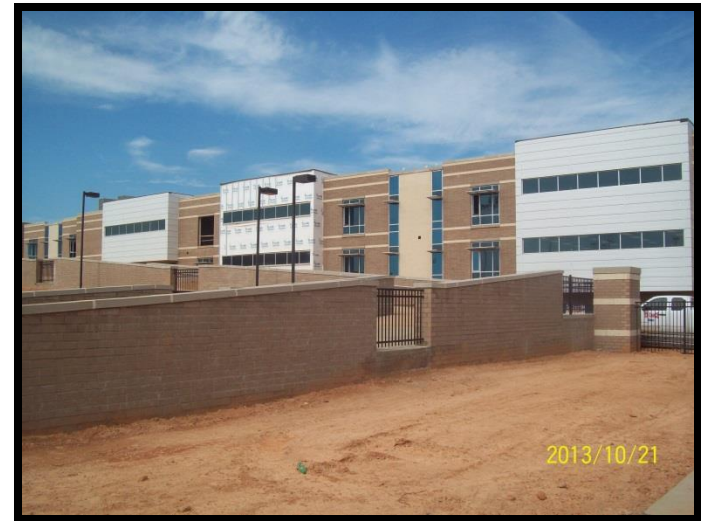
Two Story Classroom Addition from Field House
