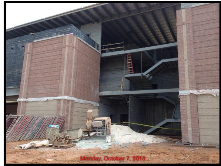
Stairs at Health Science
