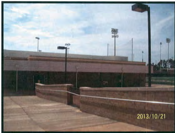
Ramps leading to Field House from Home Stands
