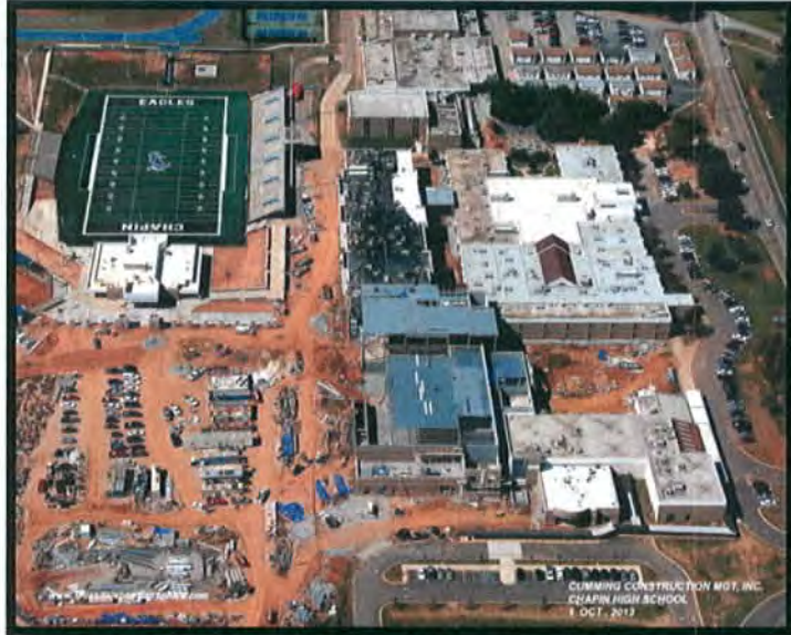
Site Aerial along Columbia Avenue
