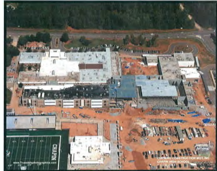
Site Aerial towards Columbia Avenue
